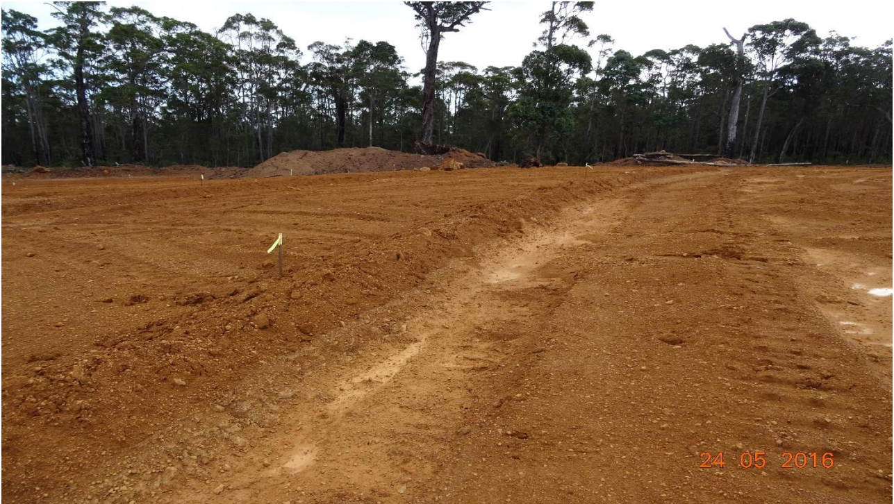
Figure 3. Contour banks used to control storm water run-off during pit preparation works.
