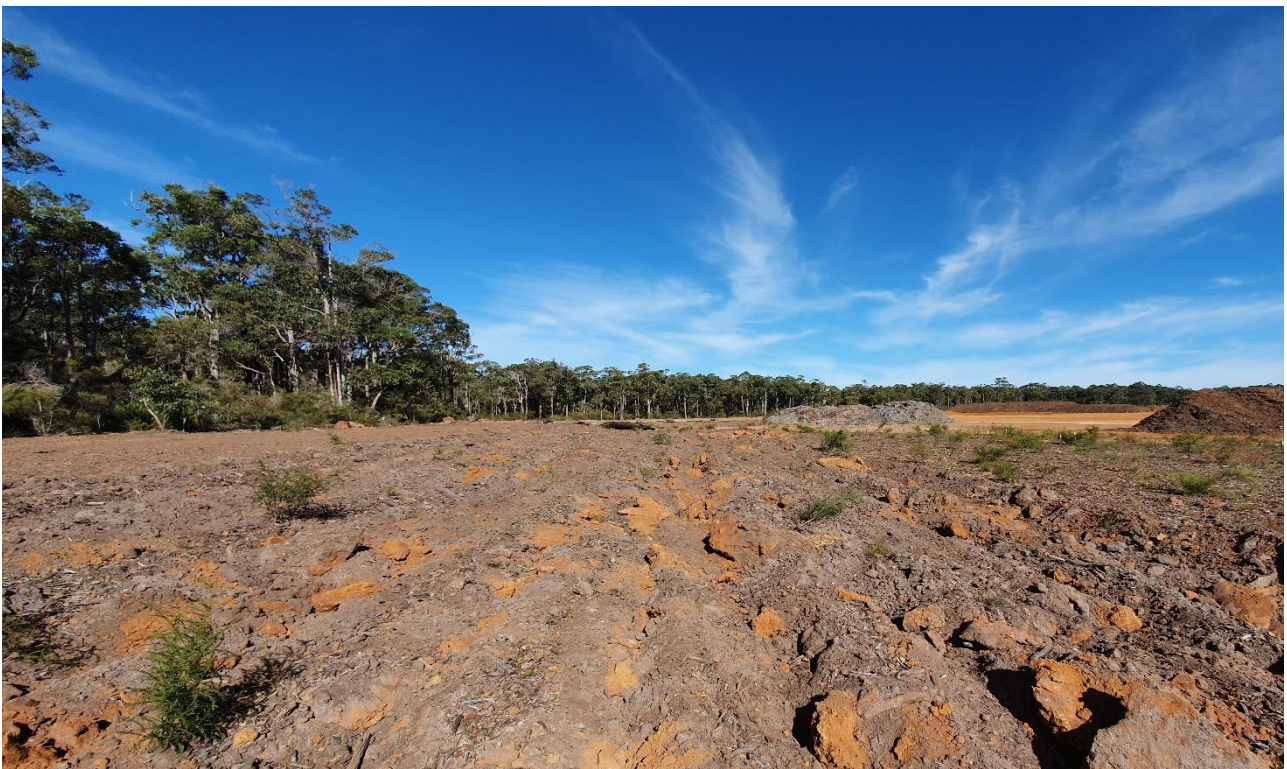
Figure 4. Pit floor deep ripped to 800mm prior to direct seeding.
