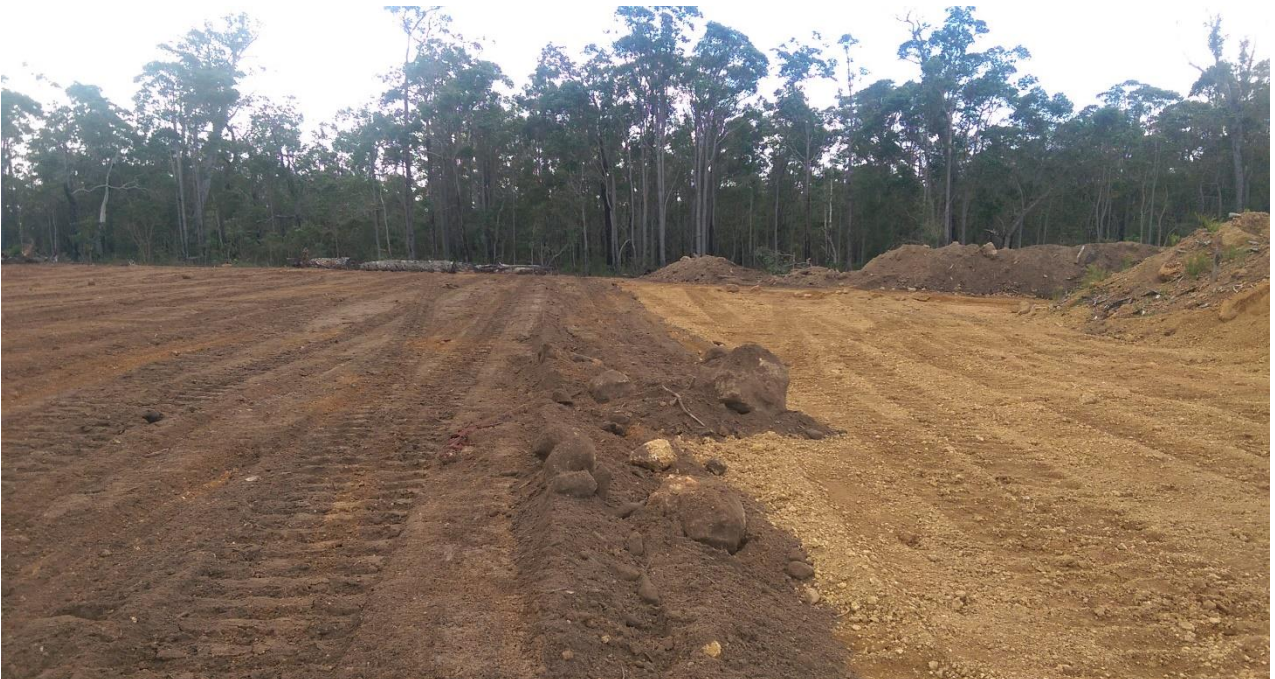
Figure 2. Top soil spread over pit floor prior to deep ripping. Habitat logs and rock near pit boundary.
