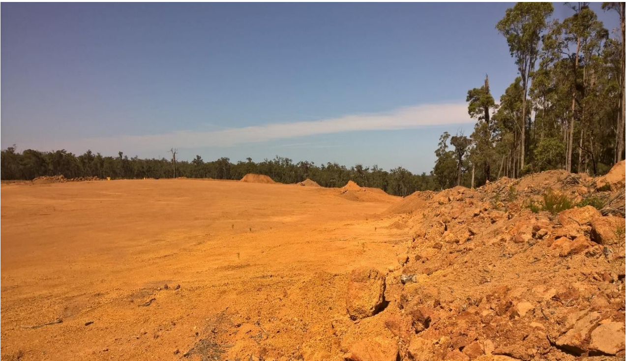
Figure 1. Typical final pit floor level with topsoil windrowed near pit boundary.
