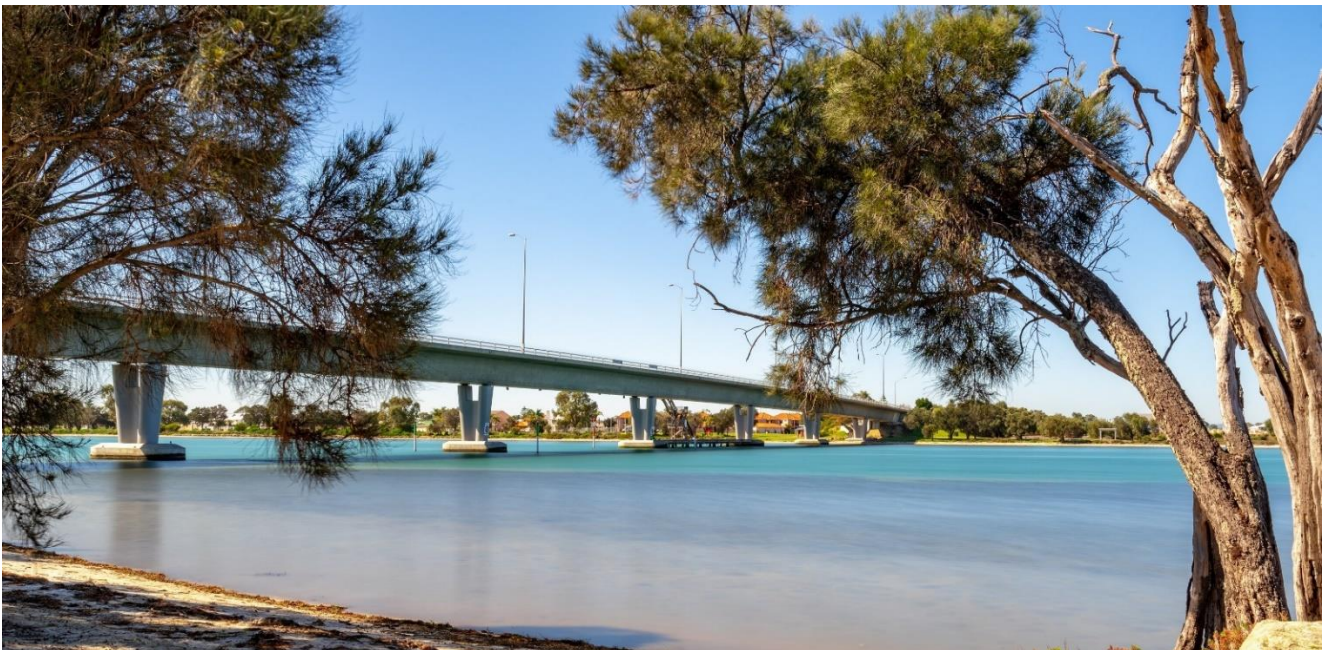
Figure 2 Existing Mandurah Estuary Bridge
