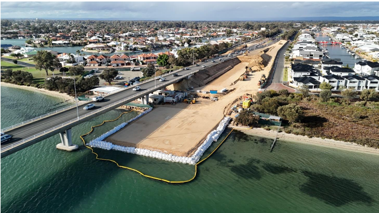
Figure 7 Reclamation Pad, on the eastern foreshore (image taken prior to sheet piling installation)
