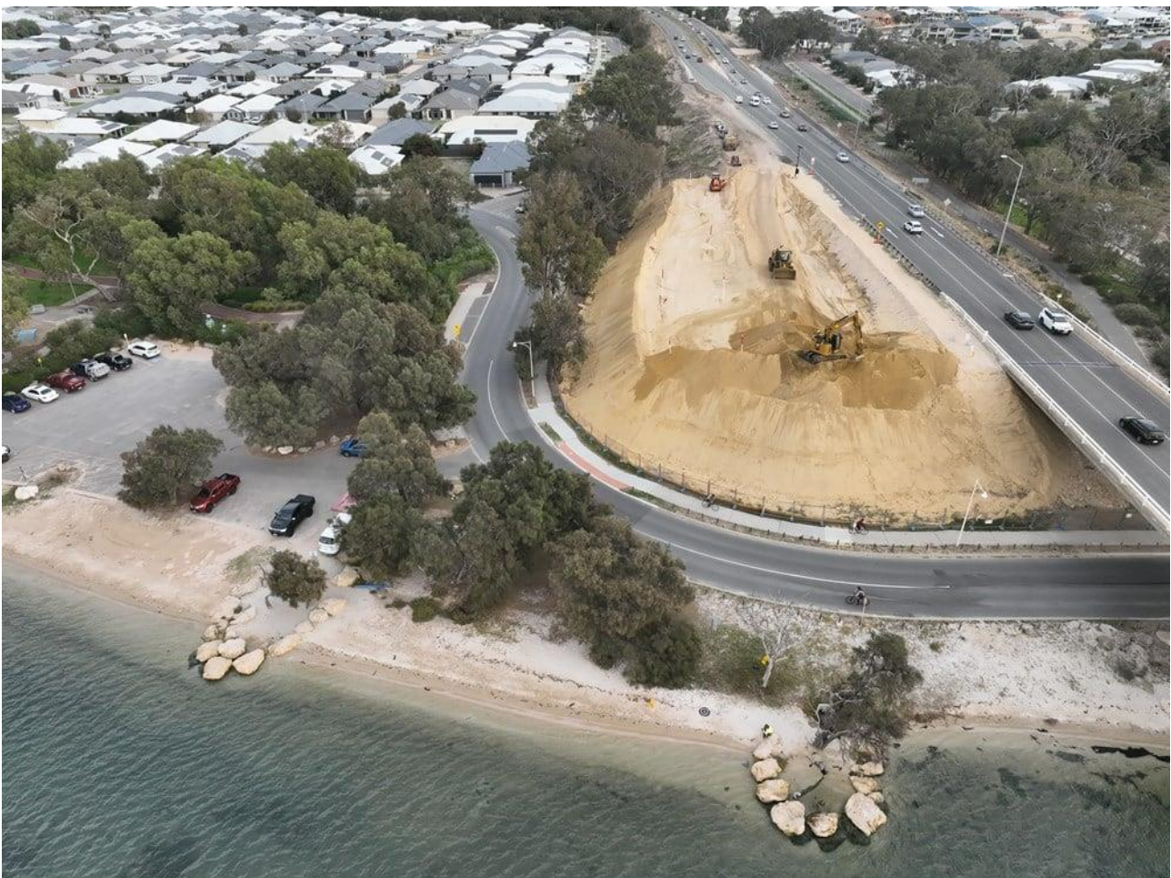
Figure 9 Aerial photograph of the preloading materials on western foreshore
