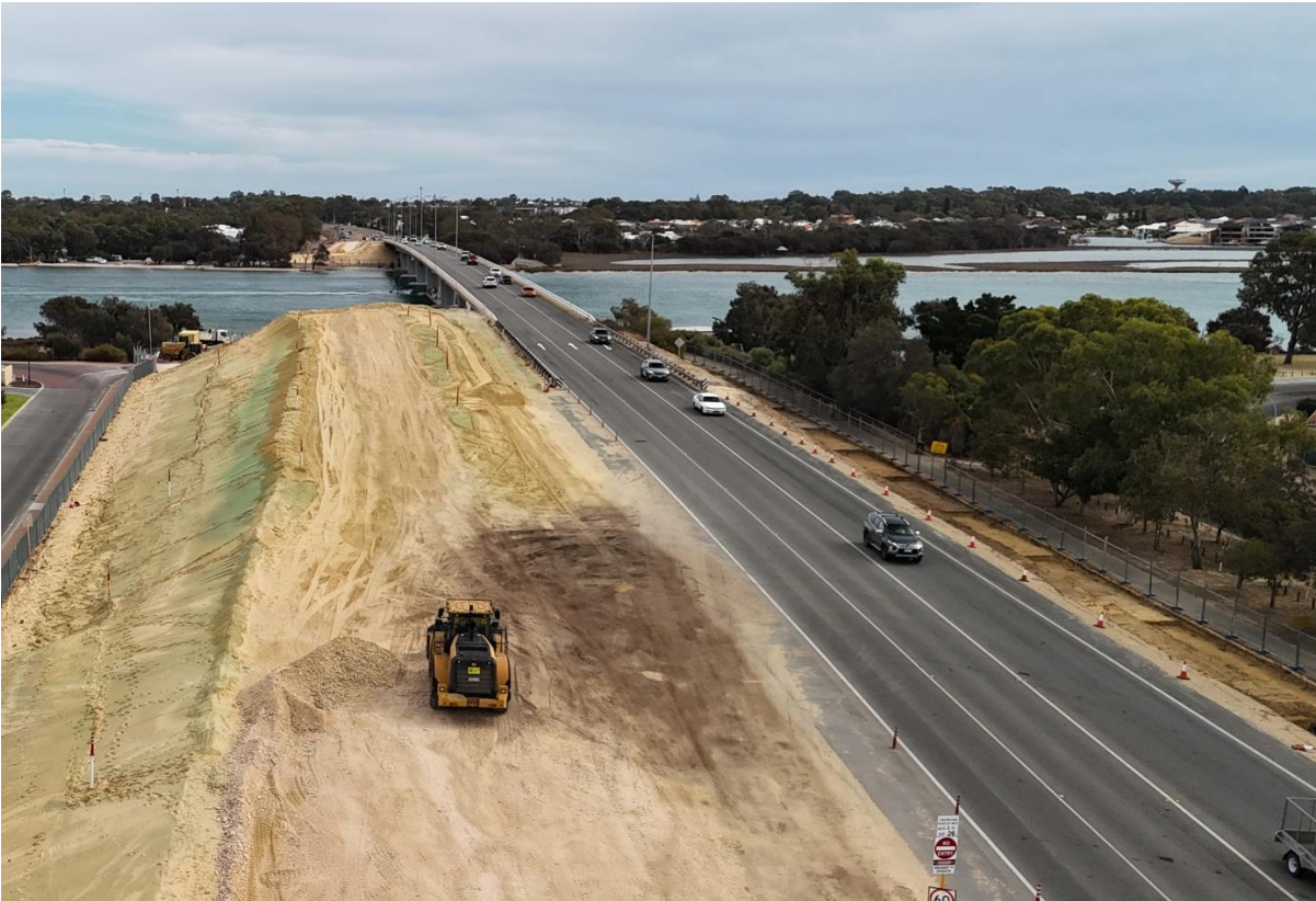
Figure 10 Aerial imagery of preloading material on the south east of the new bridge
