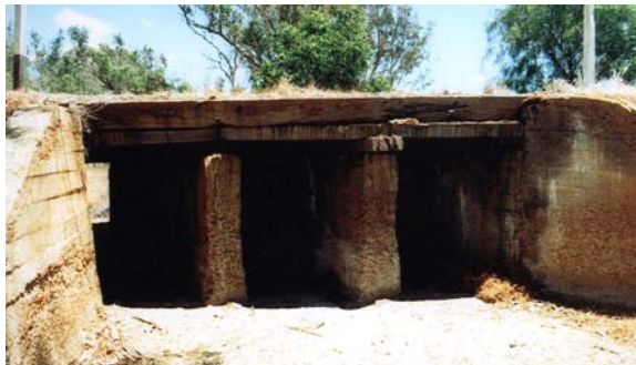
Figure 5 - MASONRY TYPE CULVERT
