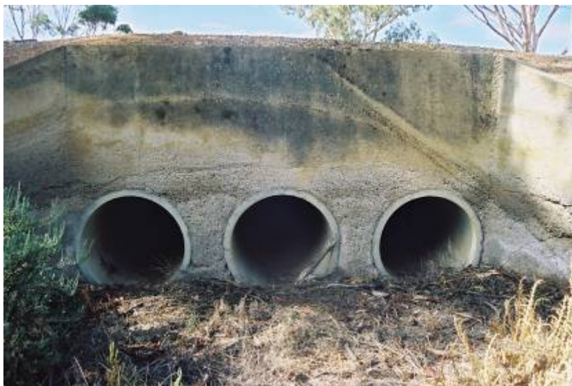
Photo 3 - CONCRETE PIPE CULVERT
