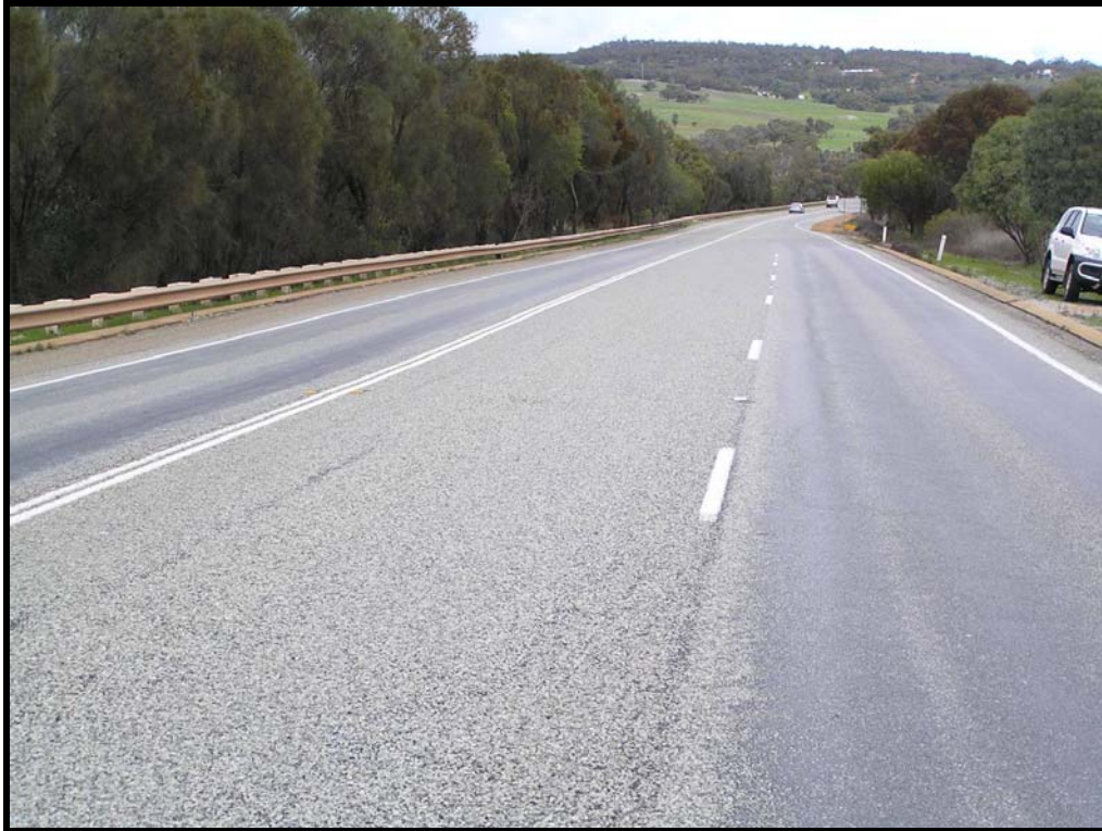
Photo 1 - TOP VIEW FROM ABUTMENT 1 END
