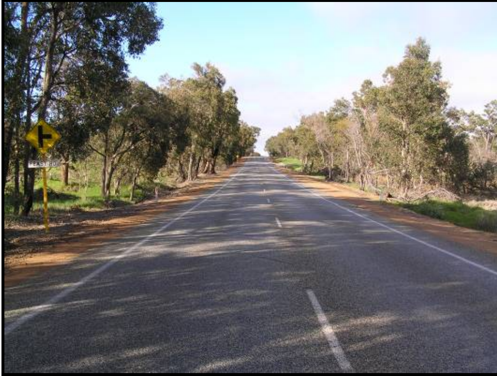
Photo 1 - TOP VIEW FROM ABUTMENT 1 END
