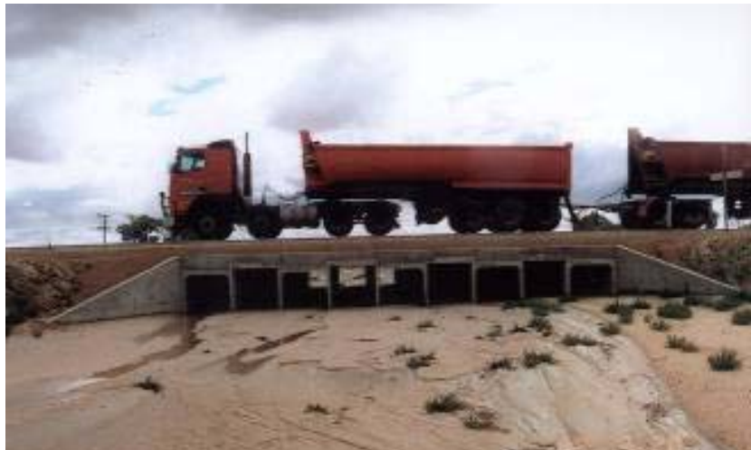
Photo 2 - REINFORCED CONCRETE BOX CULVERT (LINK SLAB TYPE)
