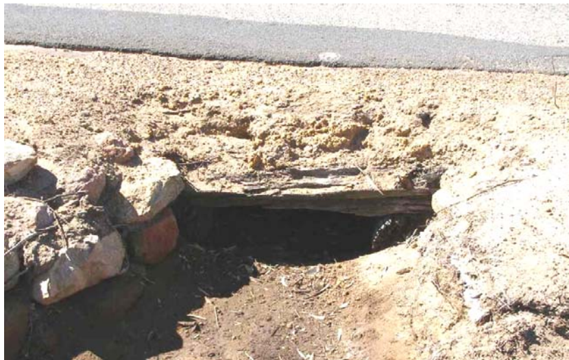
Photo 1 - TIMBER BEDLOG CULVERT
