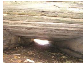
Figure 2 - BEDLOG TYPE CULVERT
