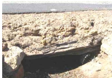
Figure 2 - BEDLOG TYPE CULVERT
