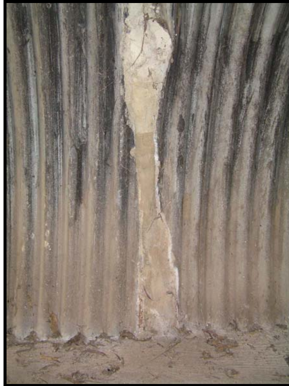
Photo 5 - TYPICAL CONCRETE PATCH AT CULVERT JOINTS
