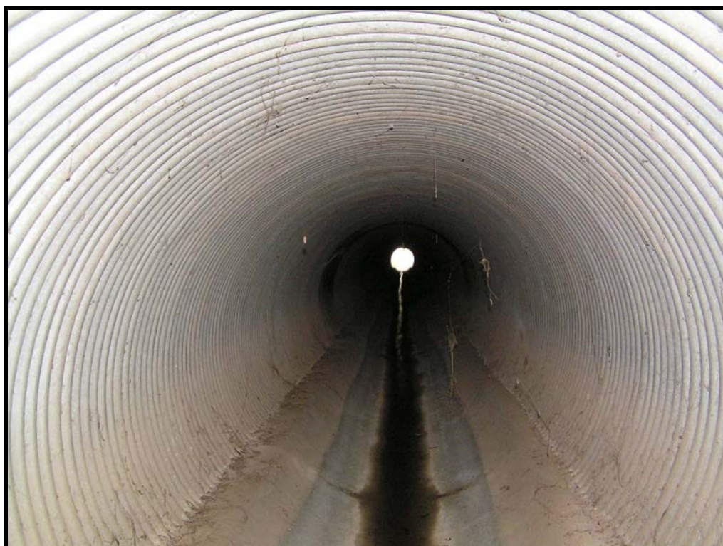
Photo 6 - TYPICAL CULVERT BARREL AND CONCRETE INVERT
