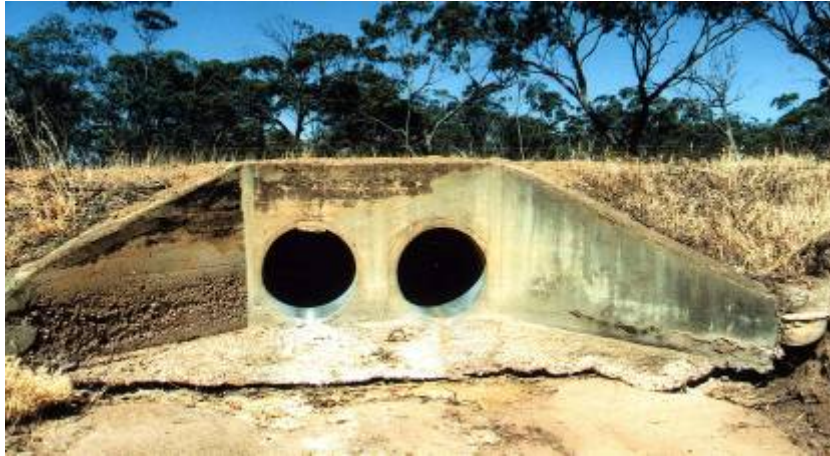
Photo 4 - STEEL PIPE CULVERT
