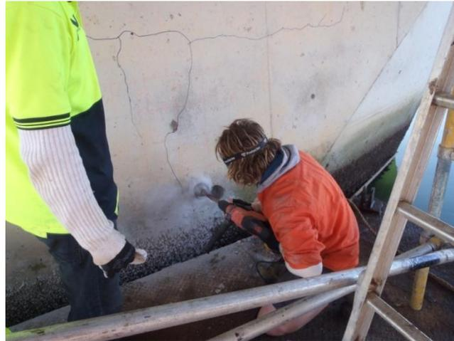
Figure 7 - Carrying out a breakout with a percussion core bit, with covermeter results lightly marked in red crayon
