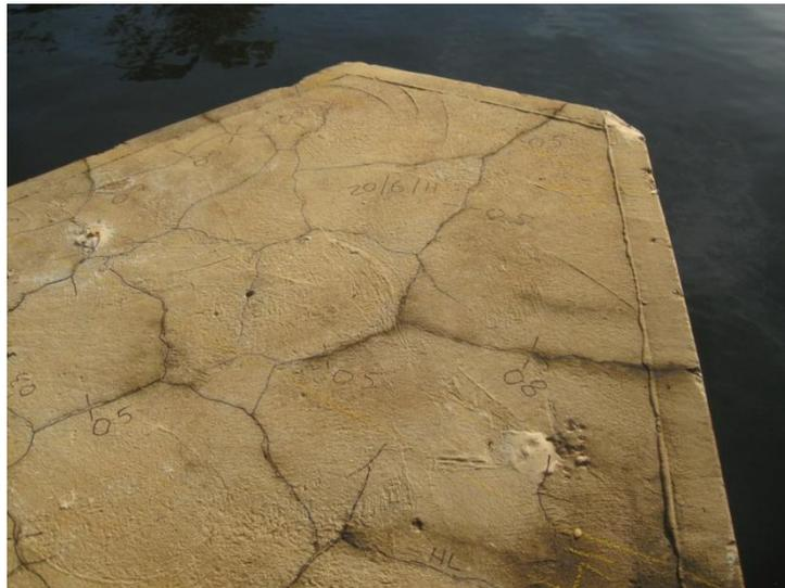
**Figure 4 - Cracking due to AAR and related dampness**
