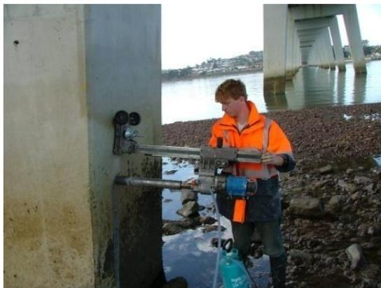
**Figure 2 – Example of taking a core**
