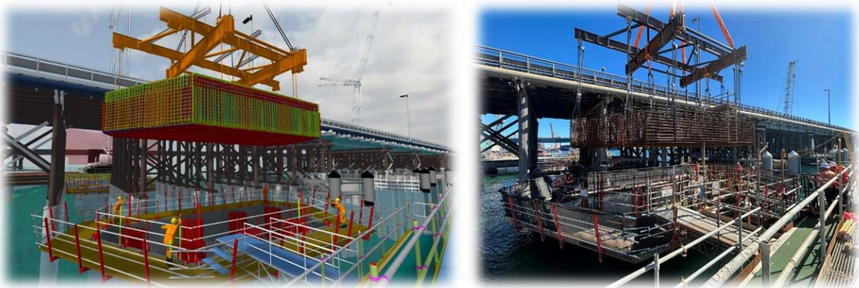
Figure 11 Digital image and corresponding photo of South-East pile cap prefabricated reinforcement cage installation
