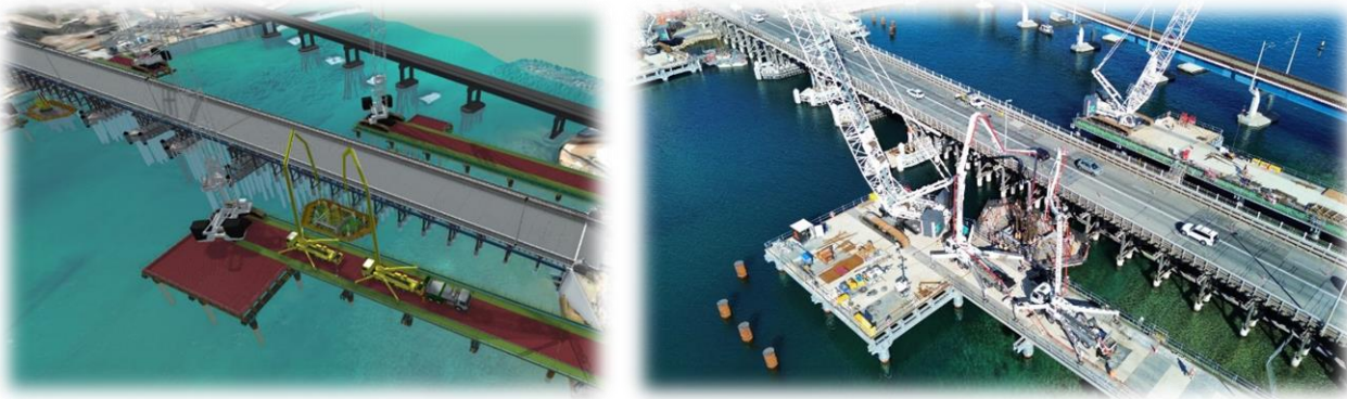
Figure 10 Digital image and corresponding photo of North-East pile cap concrete pour
