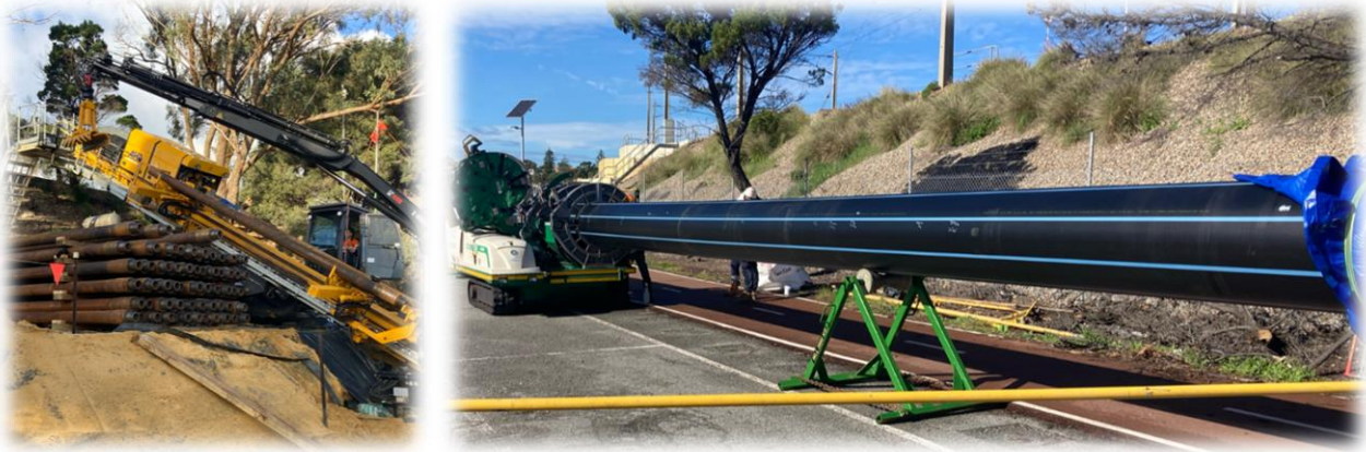
Figure 5 Horizontal Directional Drill Rig and pipe
