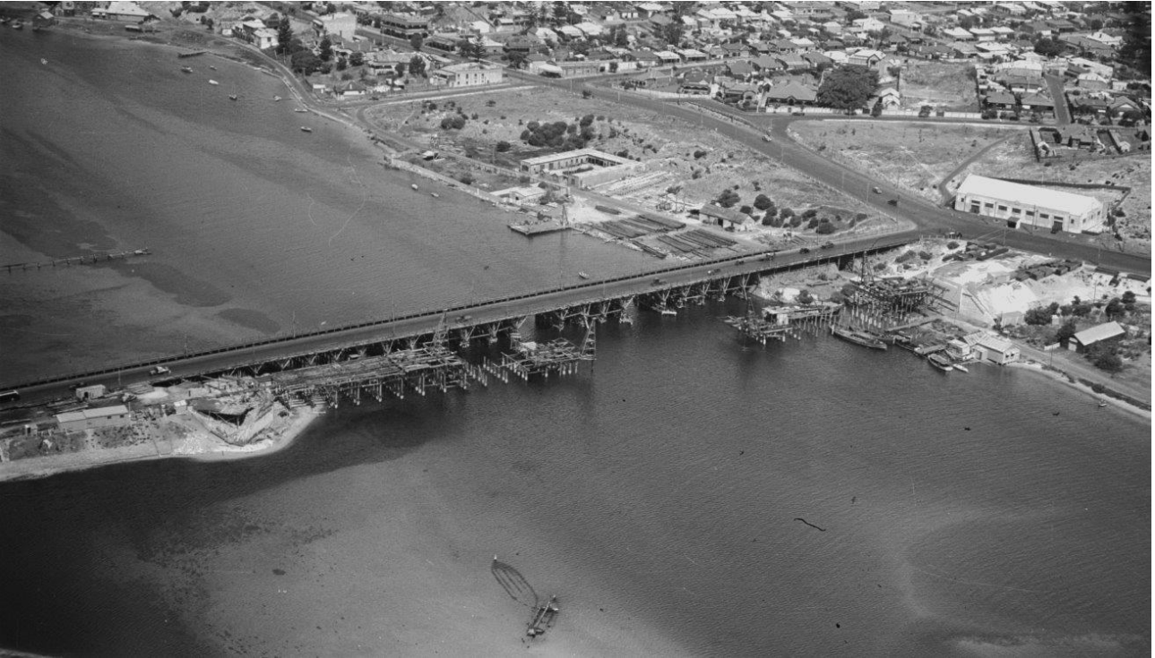
Figure 2: Construction of the Fremantle Traffic Bridge (1939)
