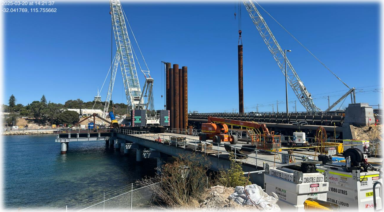
Figure 7 Photo of North-East temporary jetty with permanent piles in the background and a pile being lifted by a crane
