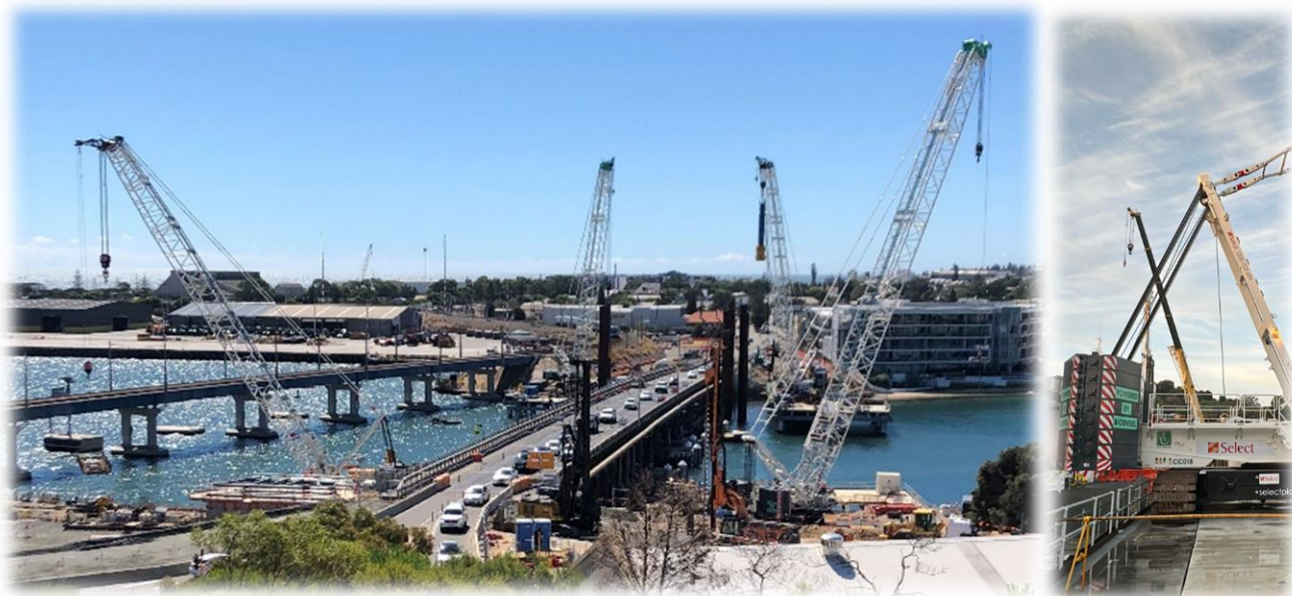
Figure 18 Temporary Jetty Cranes on project site powered by biodiesel
