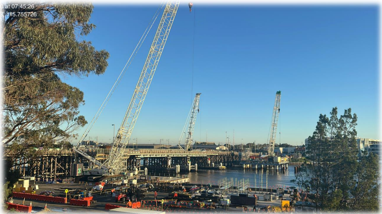
Figure 6 Photo of temporary jetties and cranes to the East of the existing bridge
