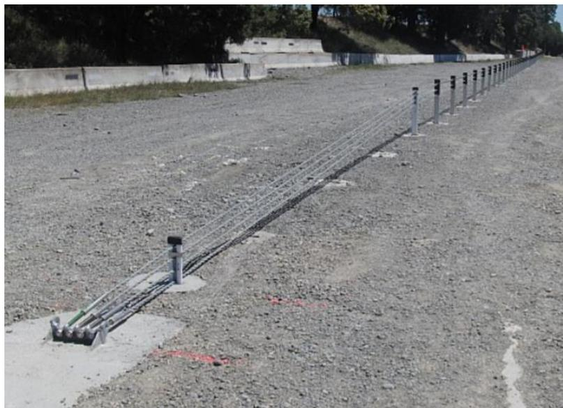
**Photograph of installed MashFlex TL3 End Terminal**
