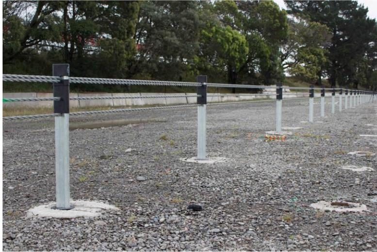
**Photograph of installed MashFlex Wire Rope Safety Barrier**
