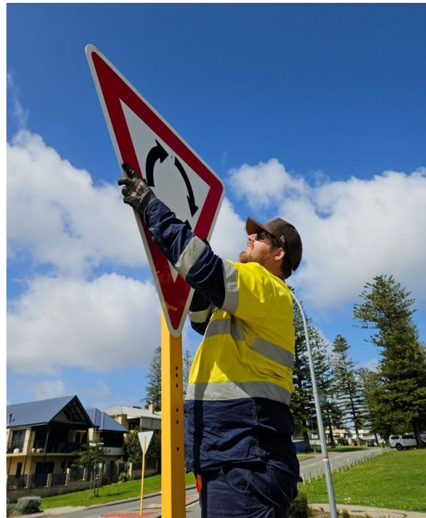
One of our Metropolitan Sign Crew in action.
