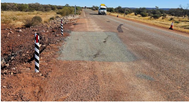
Pavement and culvert repairs on Mt Magnet Leinster Road.
