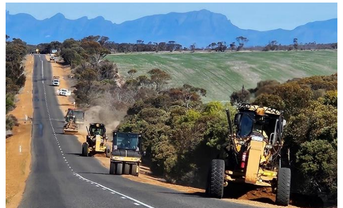
Shoulder grading underway on Albany Lake Grace Road.
