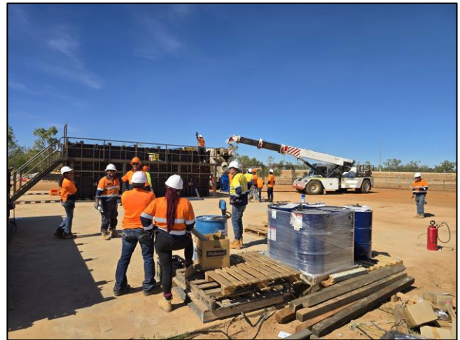
Workers on site during the box culvert pour.
