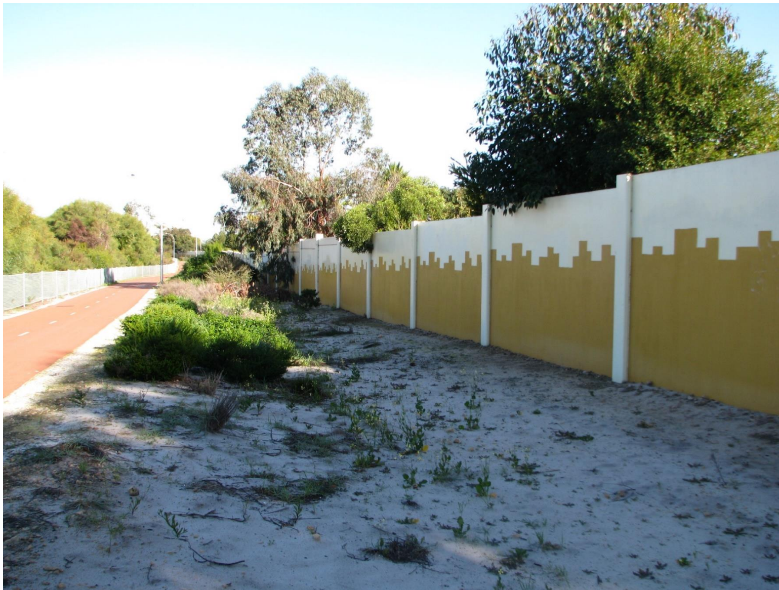
Figure 2: Site condition pre-works 2011
