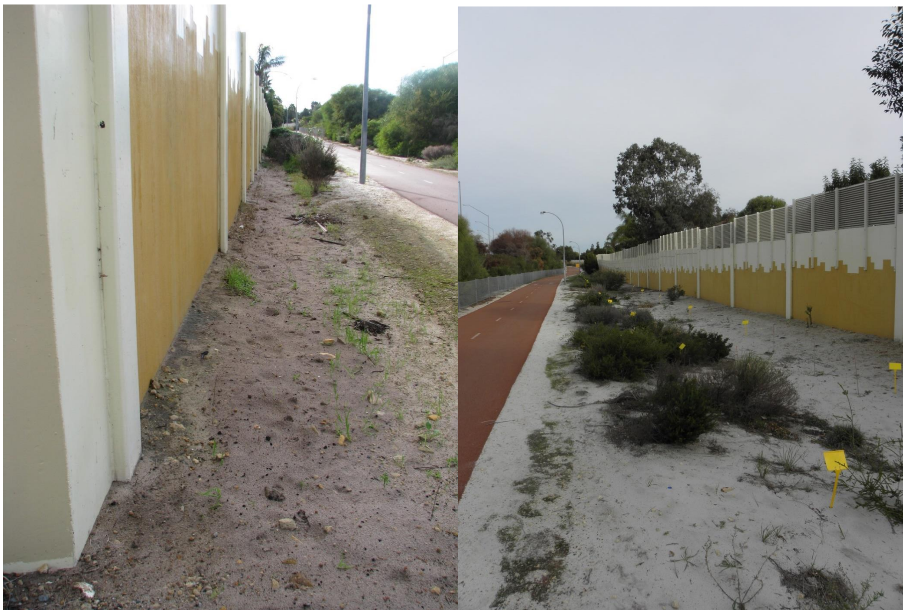
Figure 3: Site condition pre-works 2011
