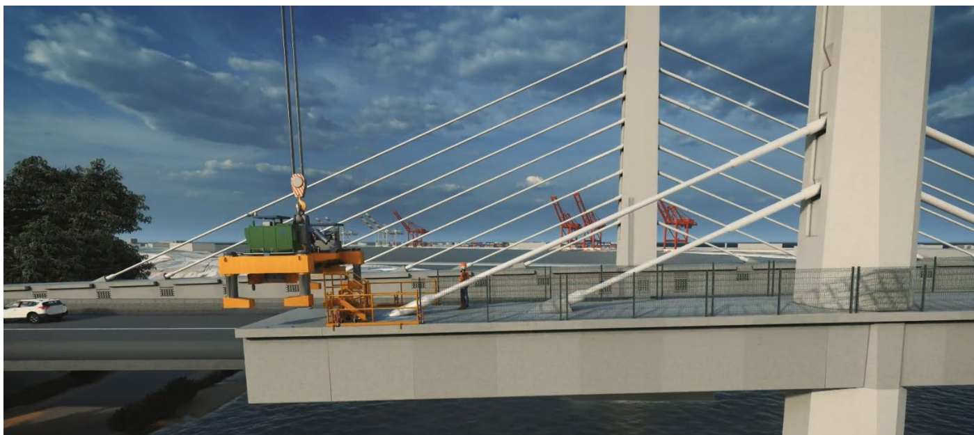
Figure 2: SLB arms rotated away and SLB lifted away from the segment.
