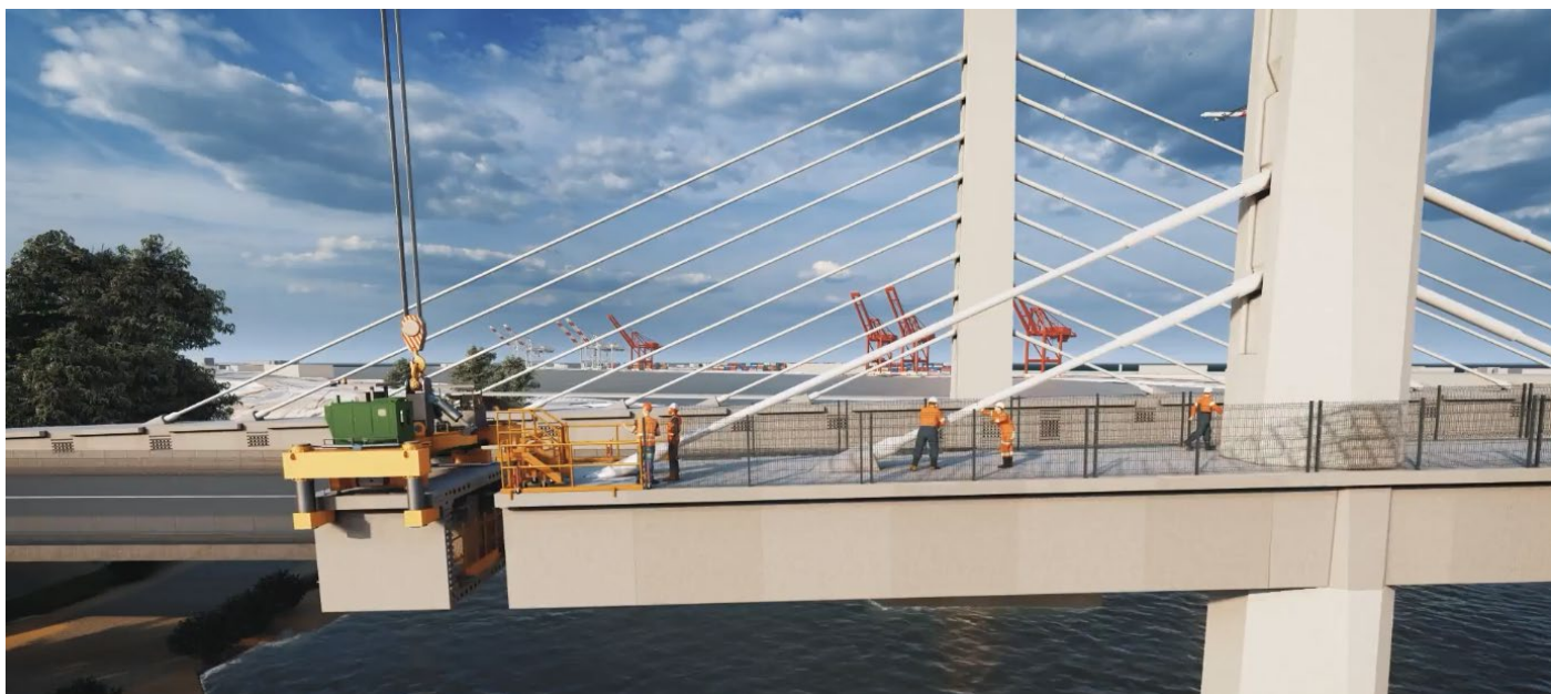
Figure 1: SLB positioning segment into place.
