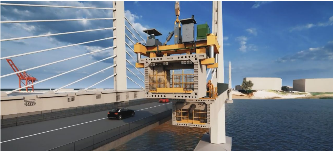
Figure 6: Segment install.
