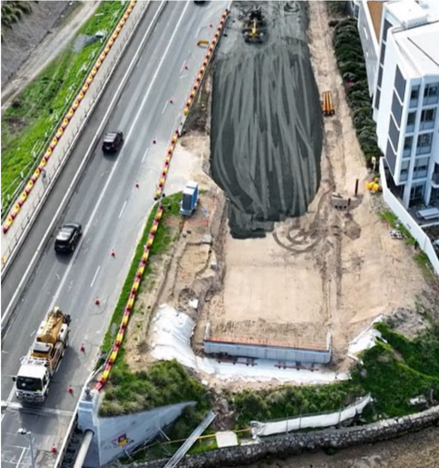
Laying basecourse for the north-east ramp.
