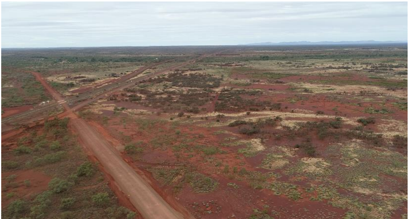
Figure 7 Northern end of Manuwarra Red Dog Highway Stage 4
