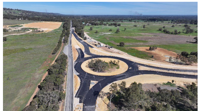
Asphalting at South Western Highway
