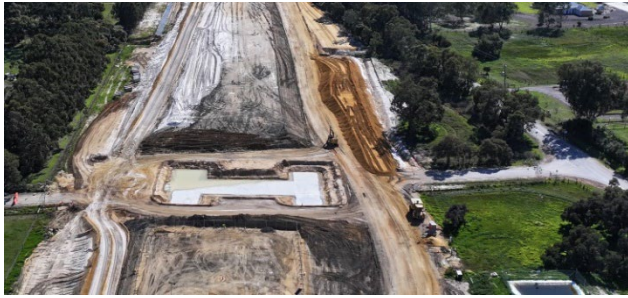
Works underway on the Gossage Road underpass.
