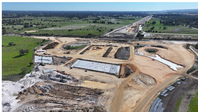
Works progressing at the Bishop Road interchange.
