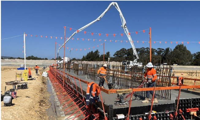
Footing for the Thomas Road bridge over Tonkin Highway.
