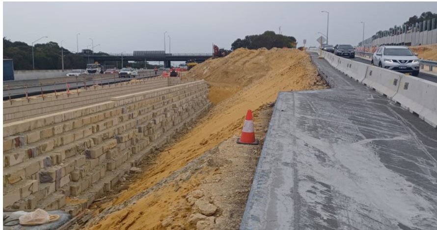
Works at the Warwick Road on-ramp incorporate a significant drainage basin.
