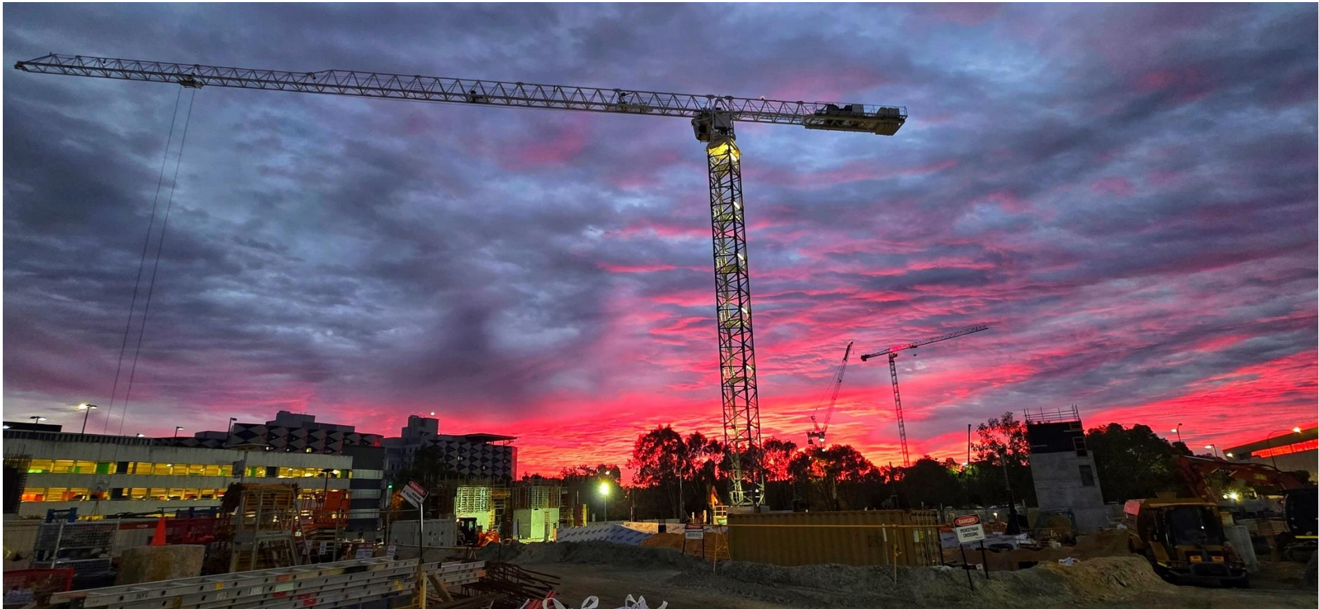
Figure 18: Tower crane erection
