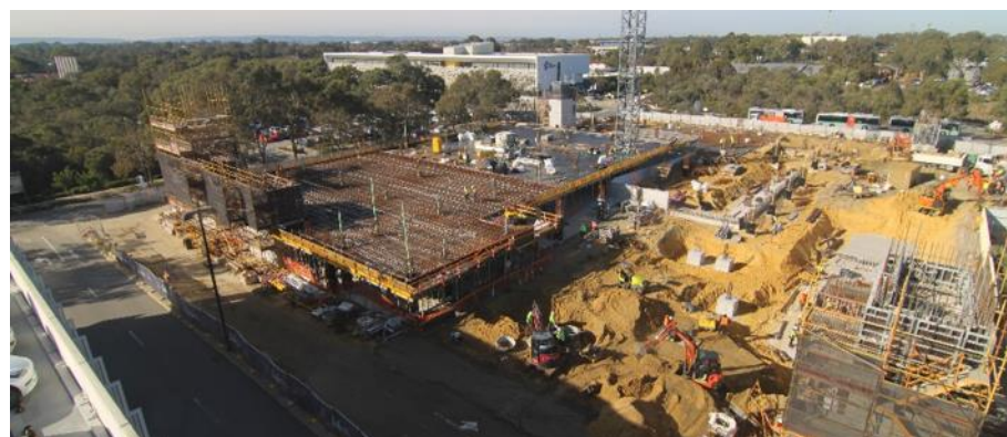
Figure 5: June 2026 construction progress
