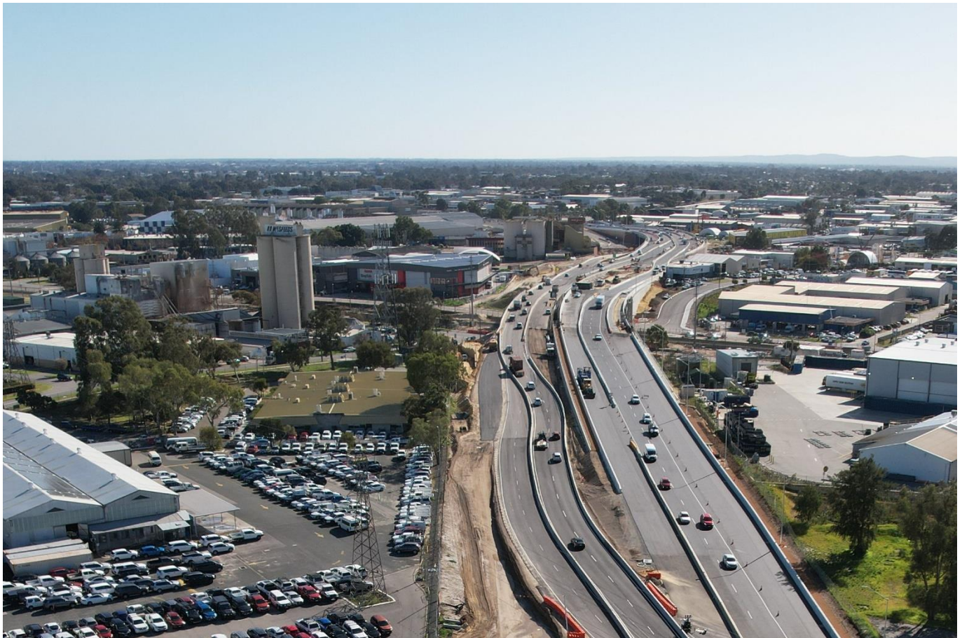
Southbound traffic on the new bridge over the Armadale rail line.
