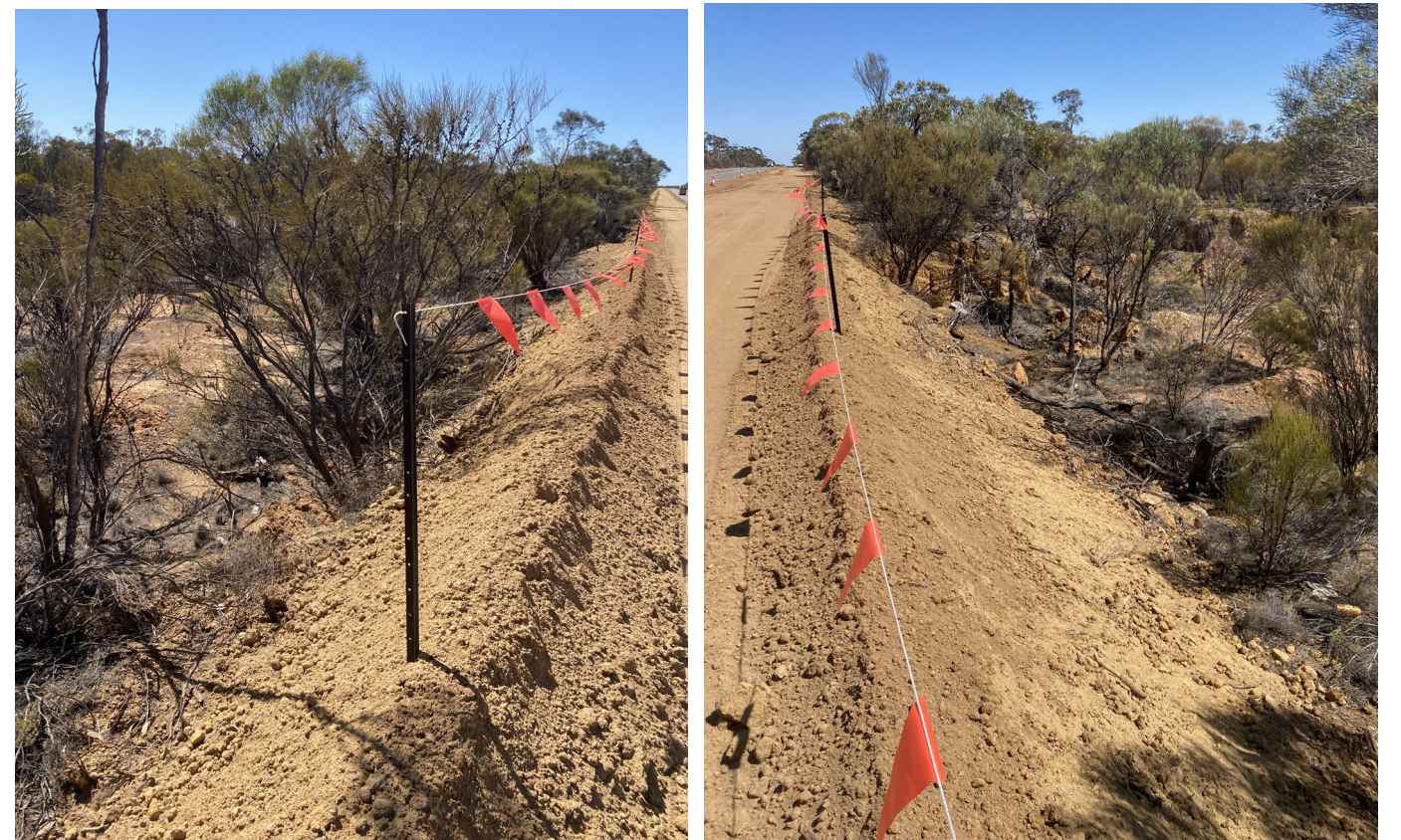
Plates 03 & 04: Eastern Clearing Area - view from edge of existing sidetrack earthworks
