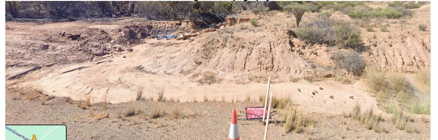
Plate 02: Proposed additional drainage modifications area looking north (Streetview). Soil heavily eroded and improvements required to formalise drainage.
