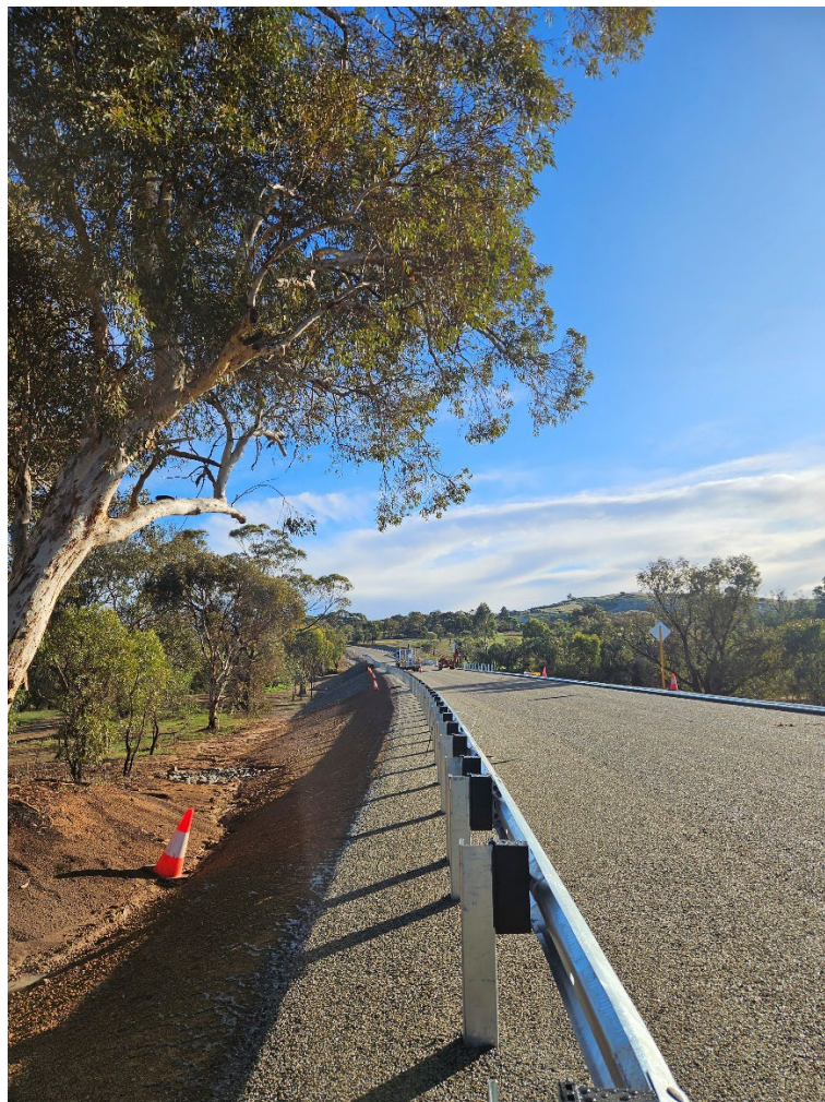
Tree looking north towards bridge post sealing works
