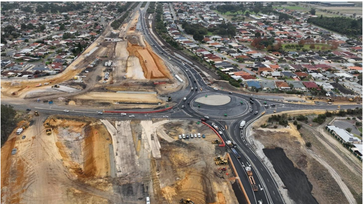
Figure 1 Construction Works – Future bridge over Altone Road.
