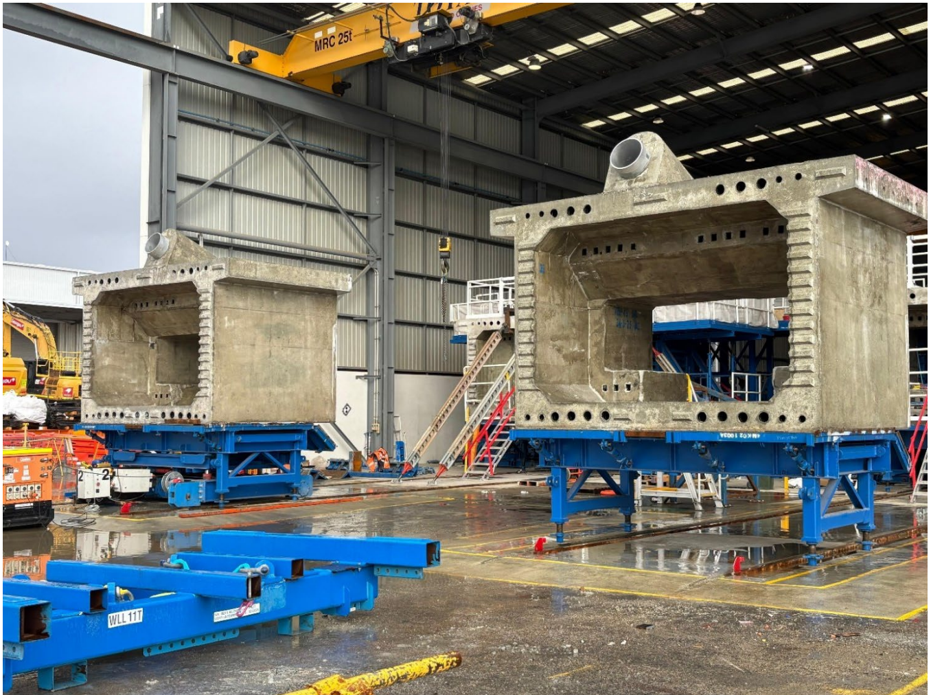
Figure 1: Edge beam segments at the precast yard.
