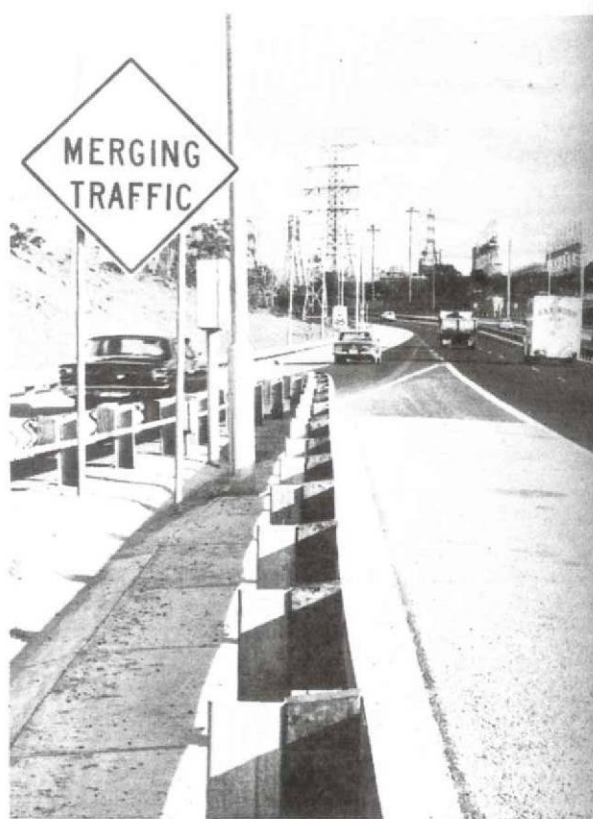
FIGURE 7. At the nose of the ramp where it joins the freeway there are wire loops set in the pavement and connected to detectors in a box which can be seen behind the traffic sign.
