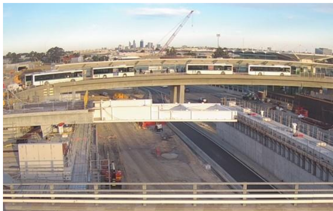
Bridge segments for the Stirling Station Bus Interchange Bridge progressing over the Mitchell Freeway.
