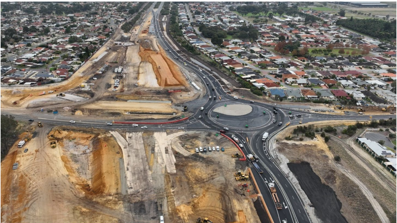
Figure 1 Construction Works – Future bridge over Altone Road.
