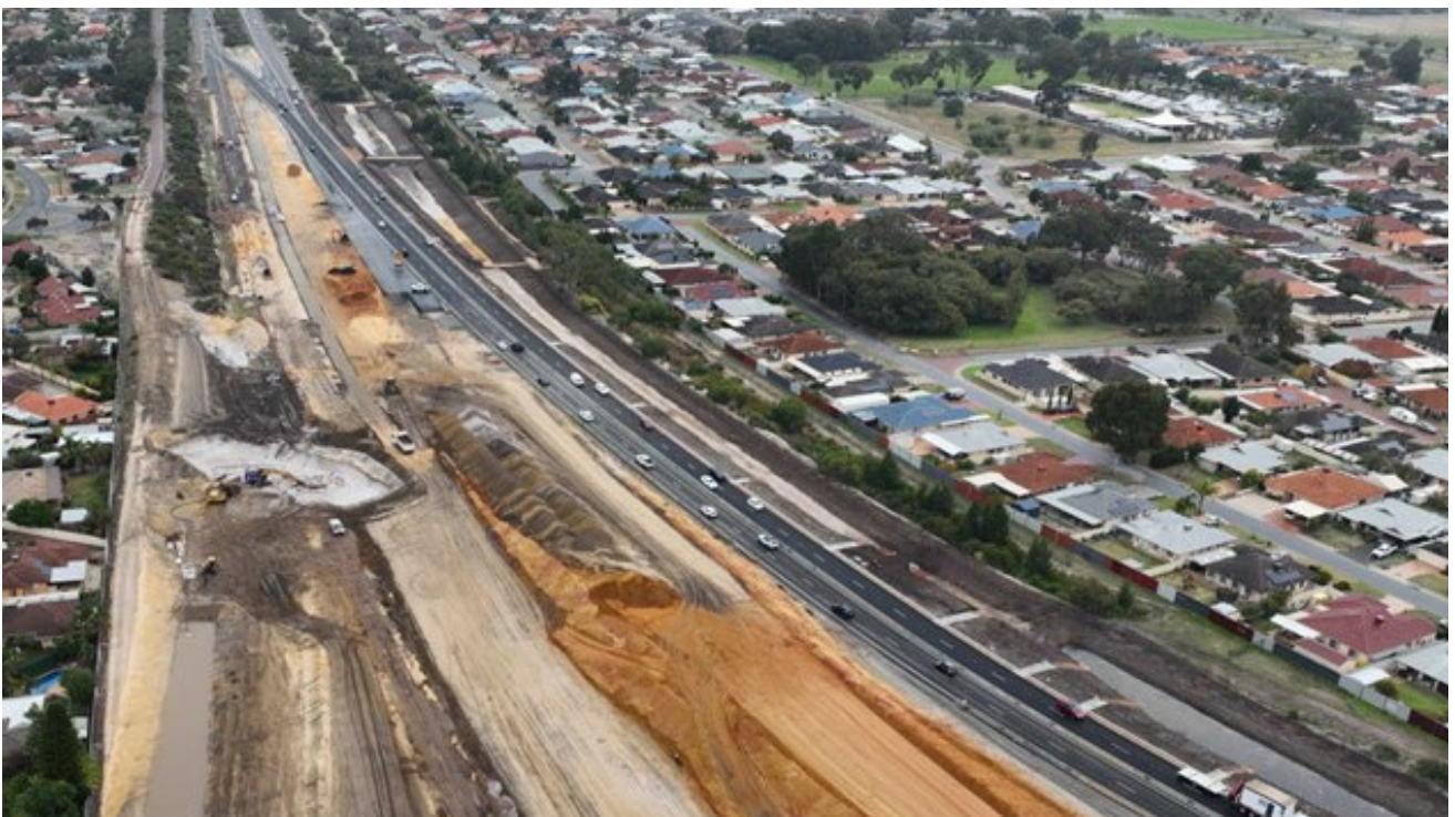
Figure 12 Mature trees retained north of future eastbound off-ramp and drainage at Reid Highway / Altone Road
