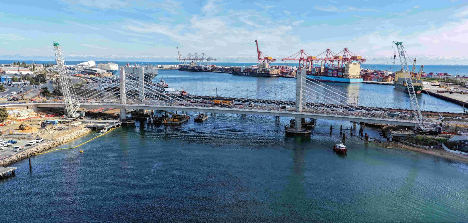
Figure 1: New Bridge Taking Shape
