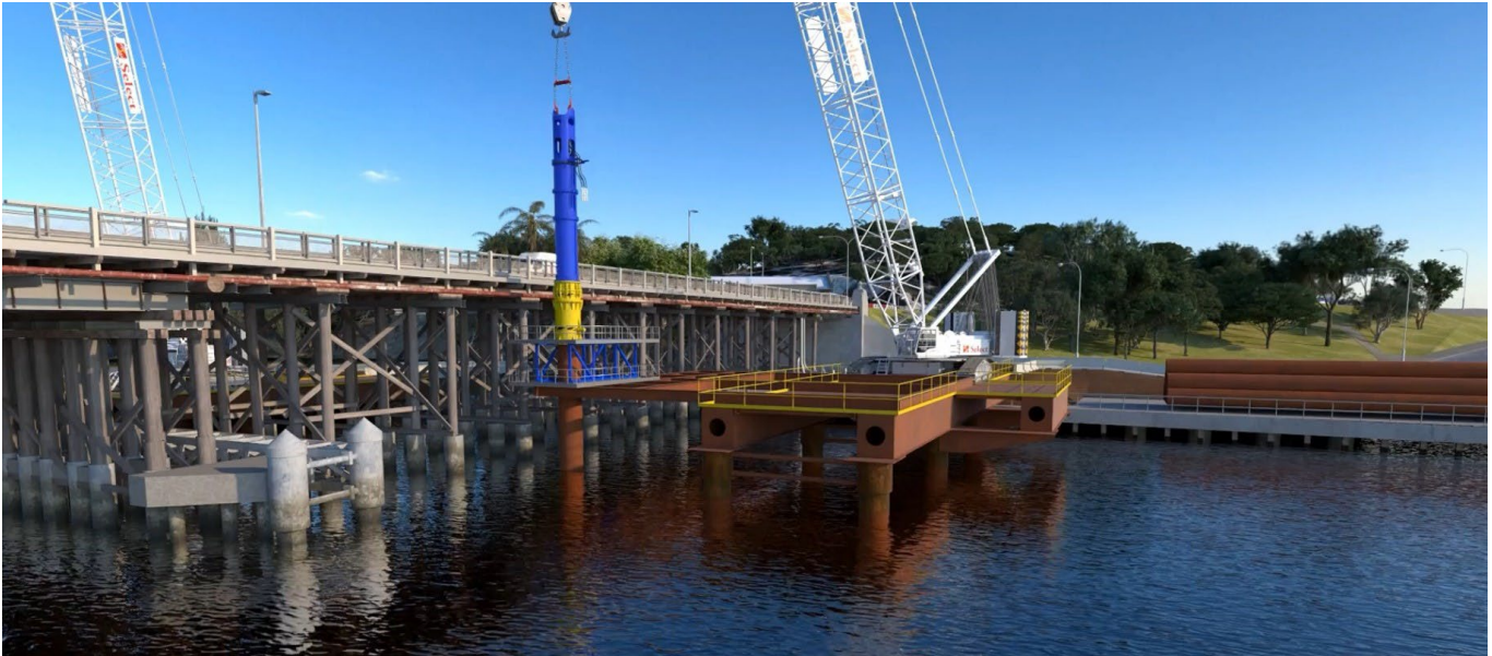
Figure 2: Piling crane in operation
