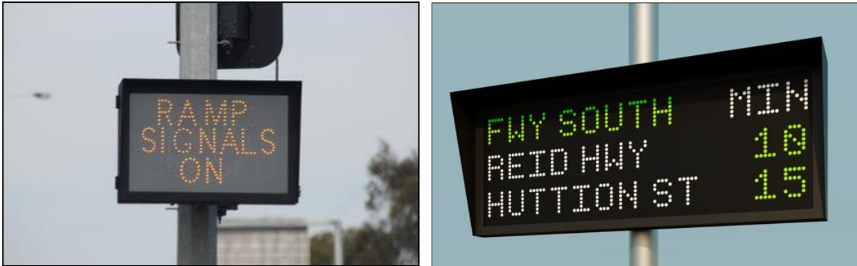
Figure 7-1: Example of an RC1 sign (left) and arterial road VMS (RC3) (right) in operation
