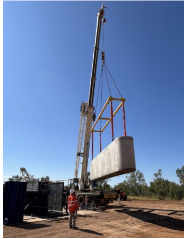
A pre-cast shell unit being moved to the work site
