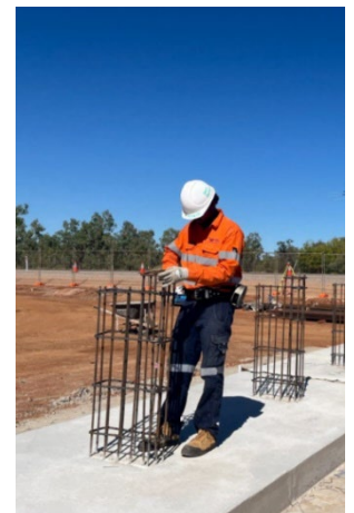
Local training - steel fixing
