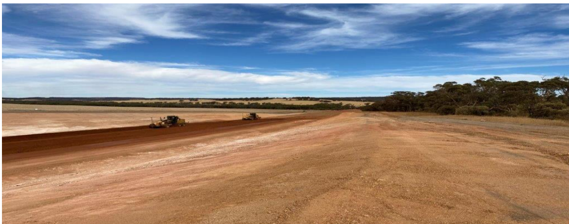
Construction between Seven Mile Hill and New Norcia
