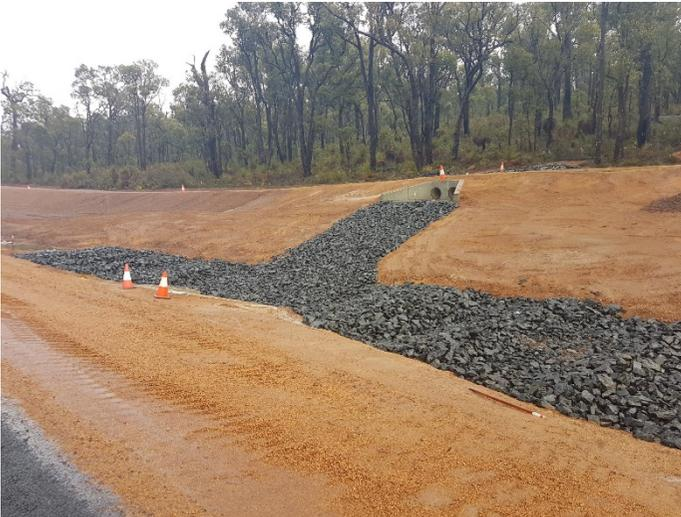
Photograph 5: Cross pollutant trap, incorporating rock protection, at the inflow point to the culvert that drains into the TEC
