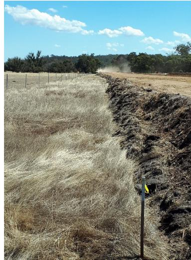
Photograph 4: Pegging of clearing line to demarcate disturbance boundary
