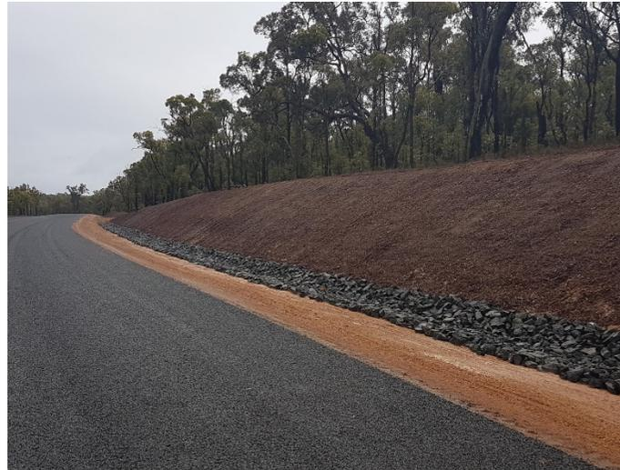
Photograph 6: Longitudinal drain scour protection
