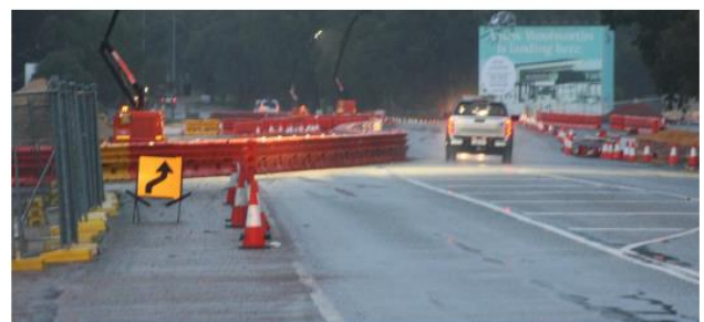
Photograph 5 – Example of northbound driver (4WD) negotiating the sub-standard taper with misleading existing lane markings on the approach to this
