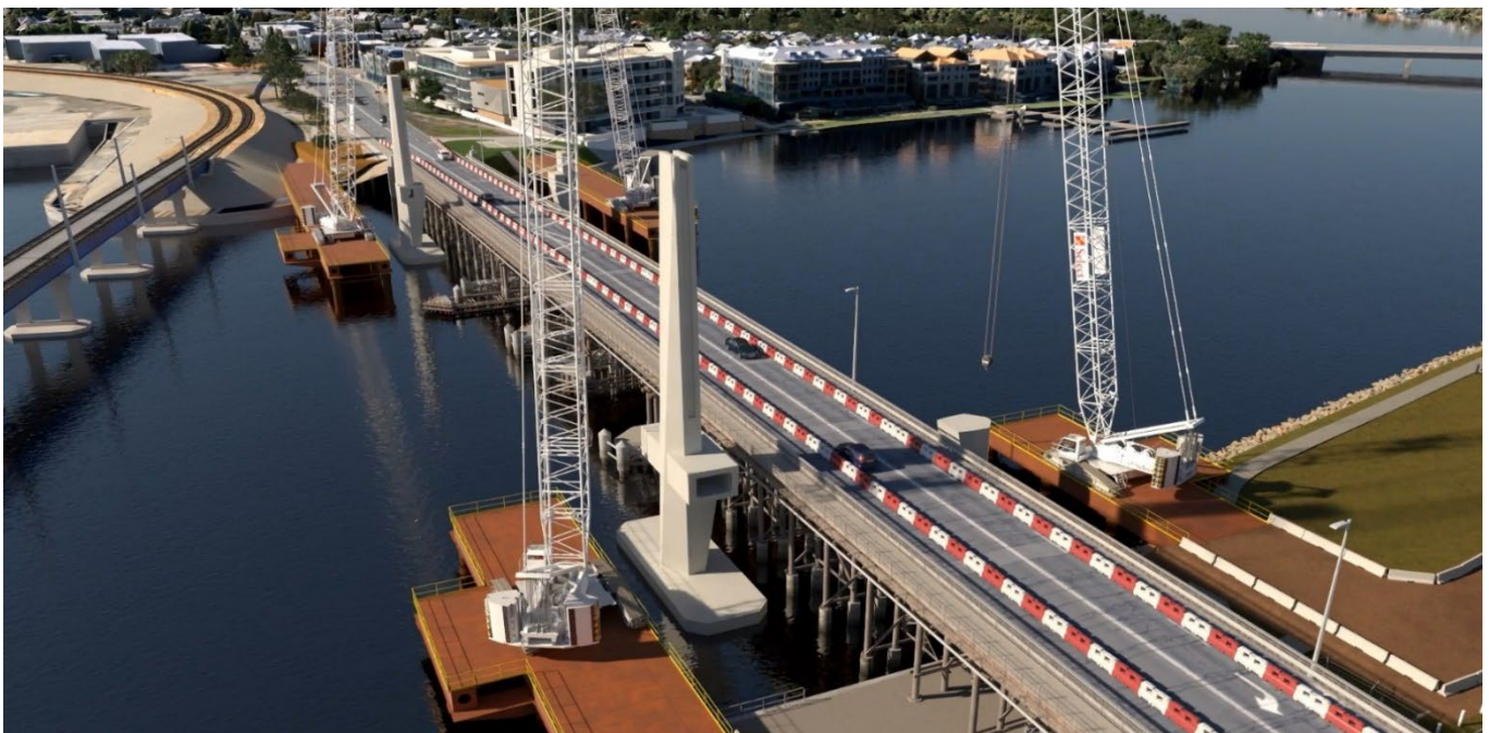
Picture 6: Completed pylons
