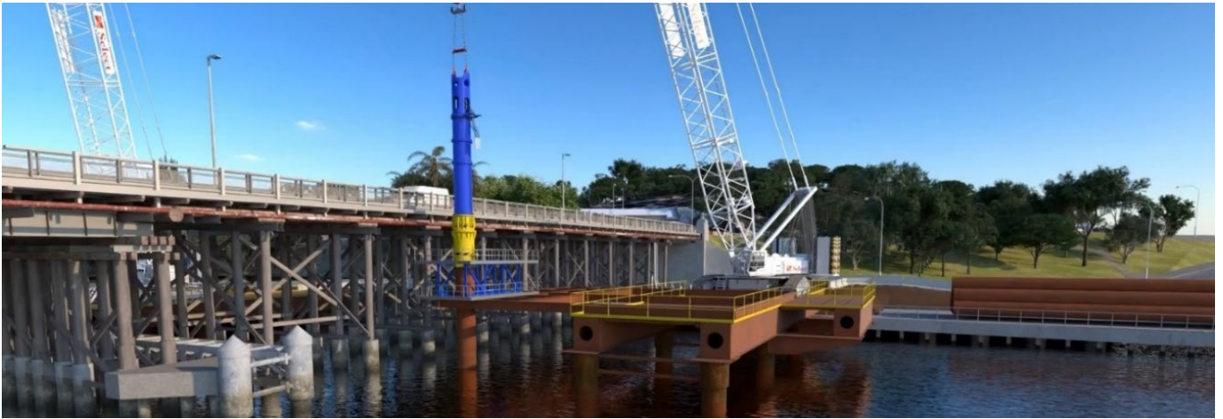
Picture 3: Hammering of piles
