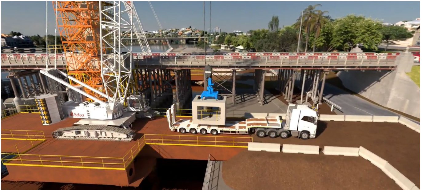
Picture 7: Edge beam segment
