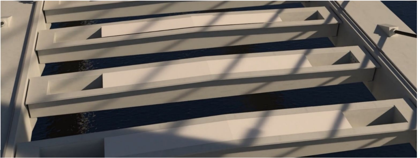
Picture 11: Bridge beams installed
