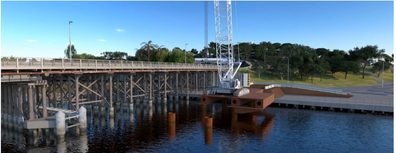
Picture 1: Crane constructing the temporary jetty
