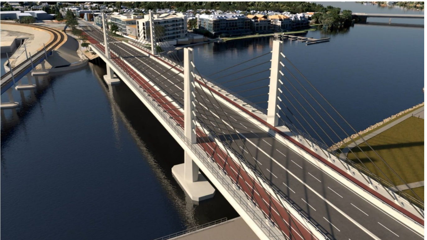
Picture 12: New bridge complete
