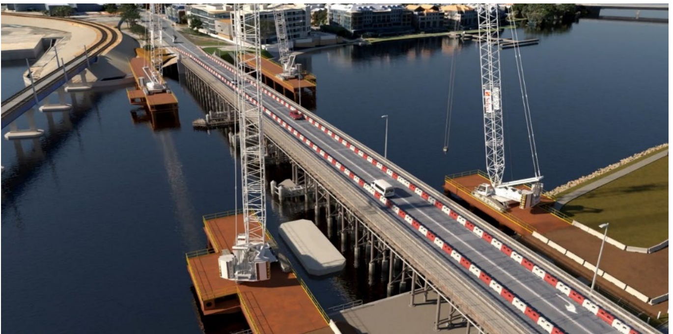
Picture 4: Pile caps complete
