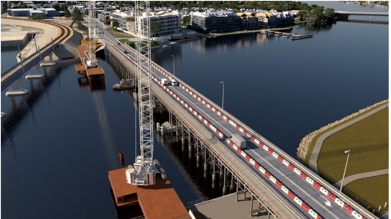
Picture 2: Two temporary jetties complete
