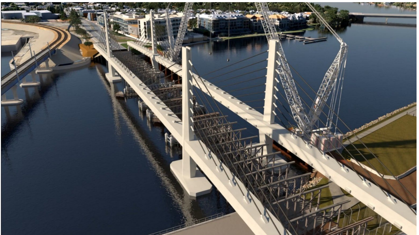
Picture 10: Removal of the existing bridge
