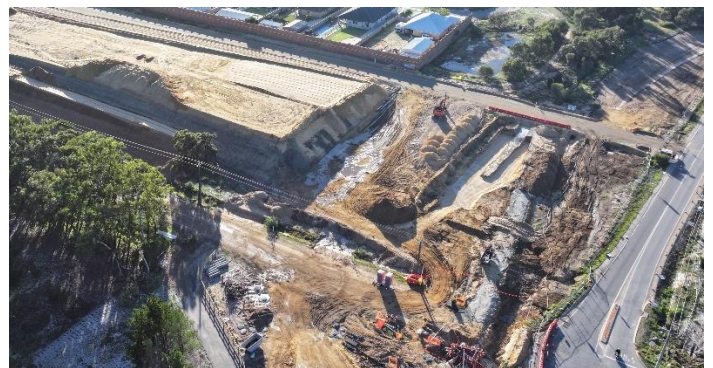
Drainage installed along Abernethy Road and bridge blinding.
