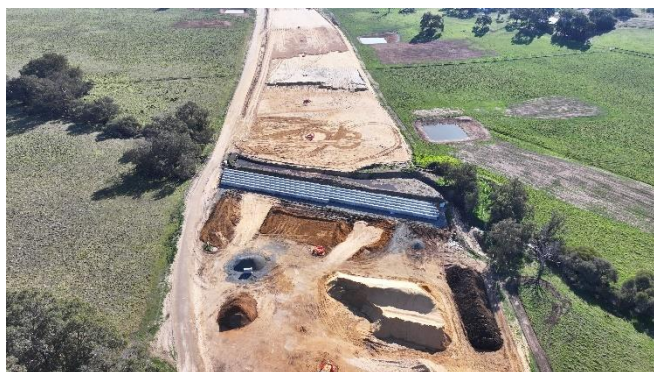
Drainage installed below the future Tonkin Highway.
