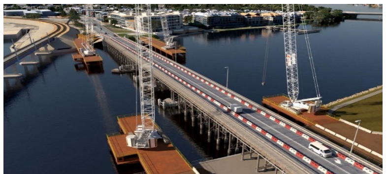
Picture 3: All four temporary jetties
