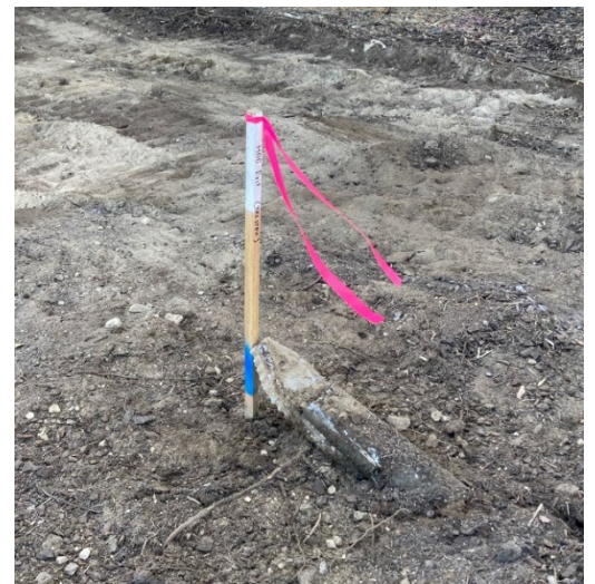
Picture 1: Telecommunications drill exit point
