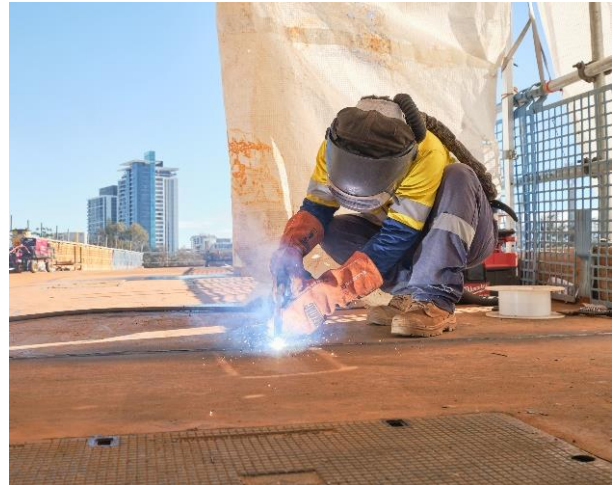
Figure 3 Welding deck modules together
