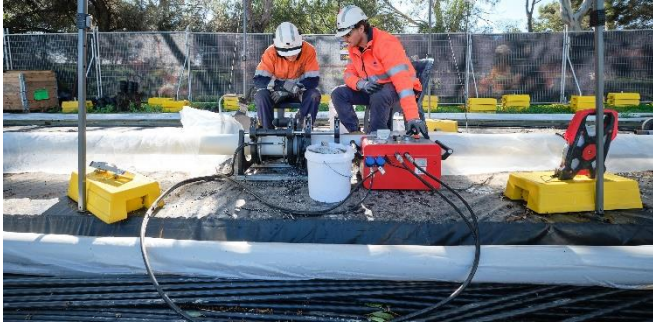
Figure 1 Preparing the cables for installation
