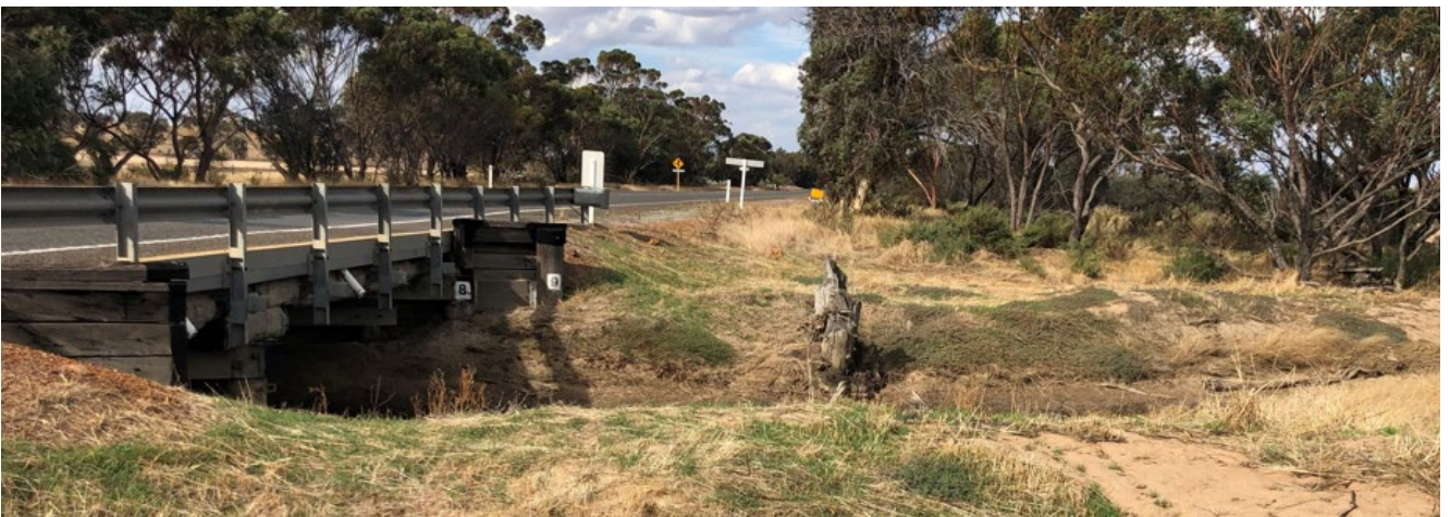
View of eastern portion of sidetrack location looking east (08-Apr-2022)
