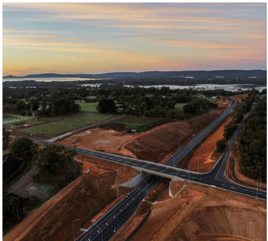
Above: New interchange connecting Menang Drive and South Coast Highway
