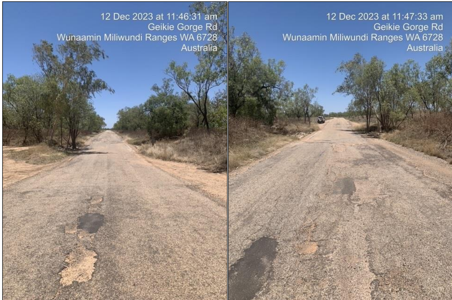
Photos 2: Maralla Creek Floodway Photos
