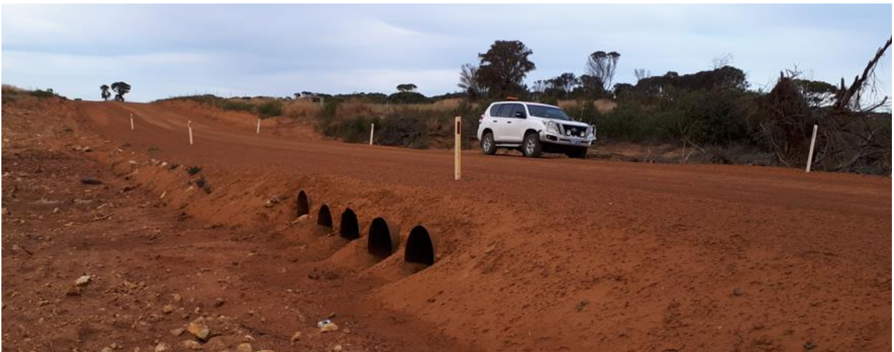
Bridge 5023A - temporary culverted crossing, looking east (June 2019)
