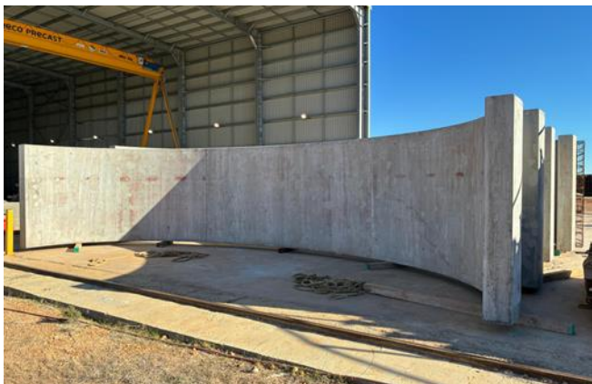
Image: Precast segments for the future underpass beneath Daviot Road.
