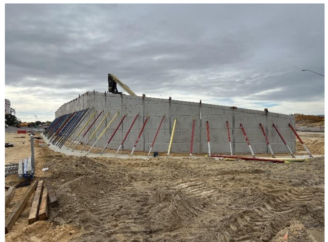
Image: Altone Road abutment wall panels during installation
