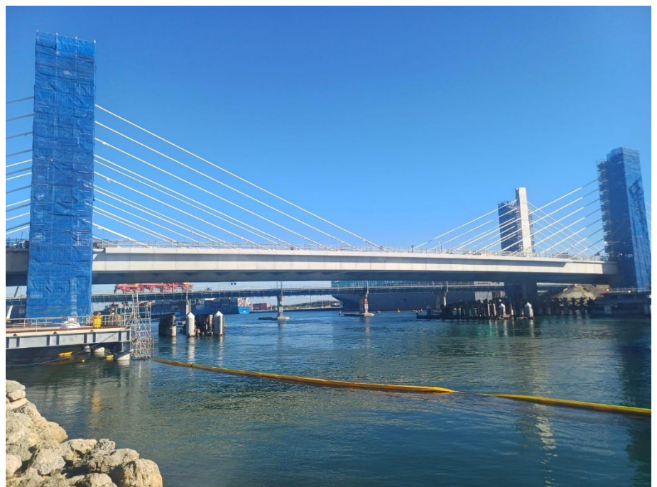
Figure 3: Navigational Channel opens up as underwater piles removed.
