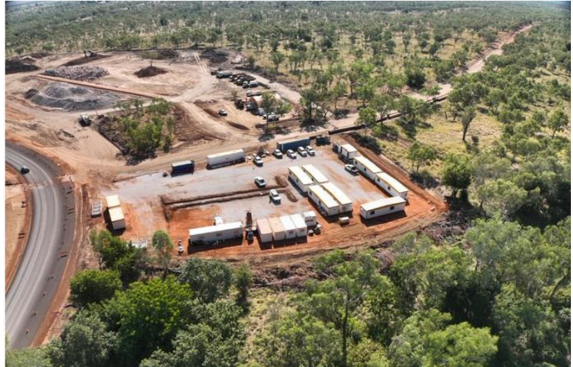
Above: Construction office in the laydown yard
