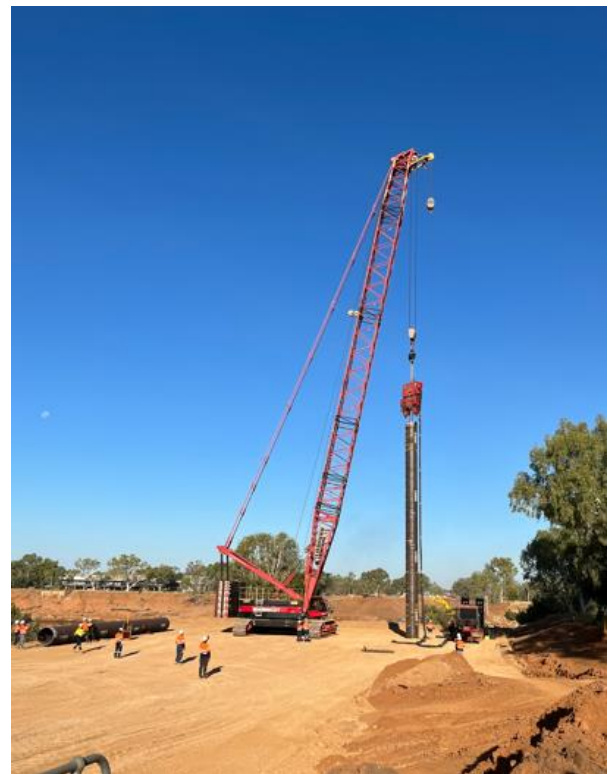
Above: Piling has started on the new bridge
