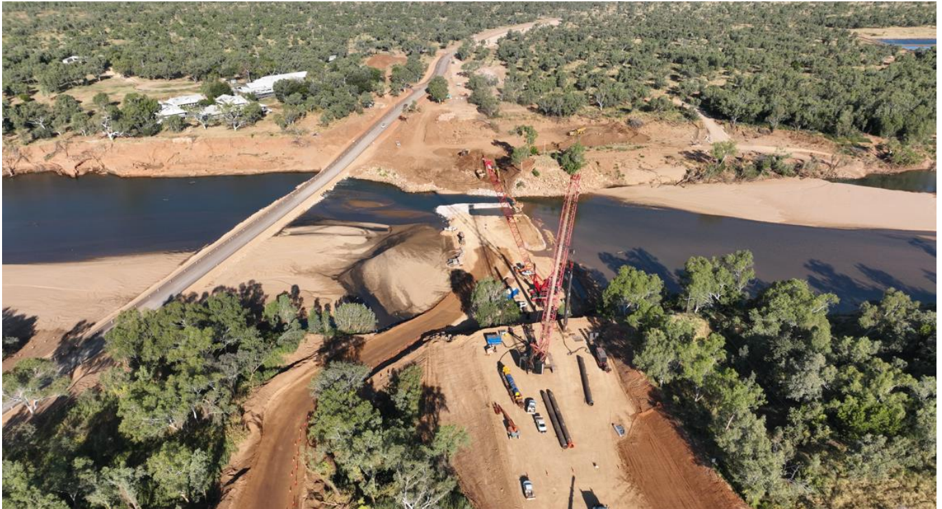
Above: Earthworks and causeway construction underway
