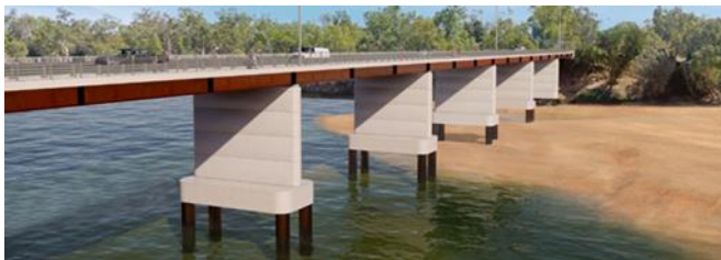
Above: Each pier consists of four piles driven into the riverbed
