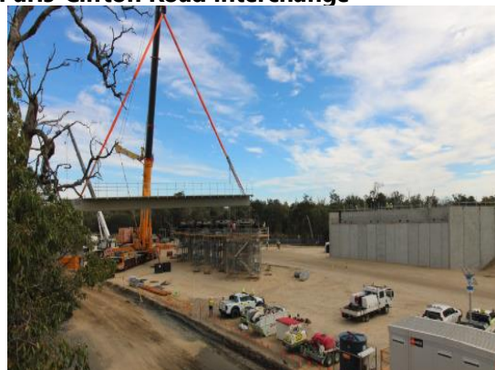
Beam install at the Bussell Highway Y-interchange
