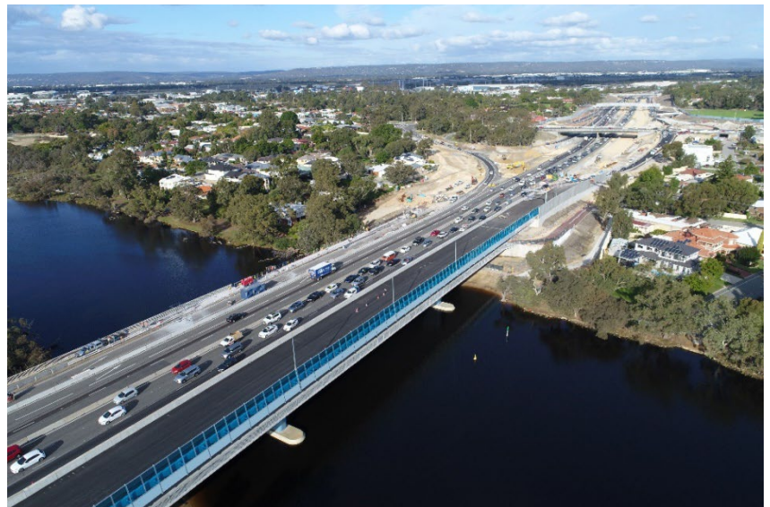
New lanes over Redcliffe Bridge
