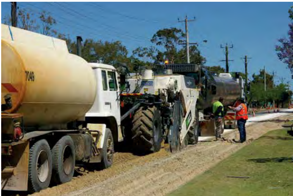
Figure 11: Foamed bitumen stabilisation, single pass mixing operation.
