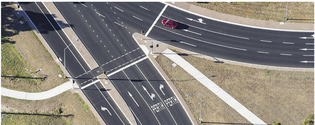
Figure 8-7: Advanced Destination Pavement Marking (Eelup Rotary, Bunbury)
