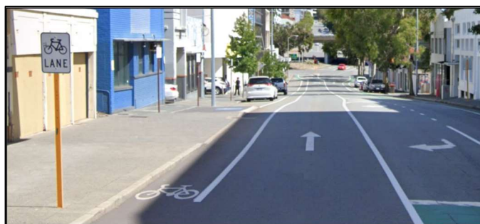
Figure 6.15 Exclusive bicycle lane signed with R7-1-4 sign and bicycle pavement symbol (Murray Street, Perth)
