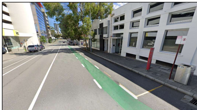
Figure 6.7 - Application of green surface treatment where bicycle lane interfaces with bus stop (Murray Street, Perth)
