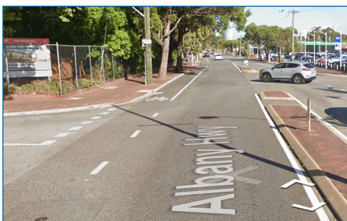
Figure 6.14 - Application of bicycle pavement symbol to sealed shoulder in an urban environment (Albany Highway, Victoria Park)
