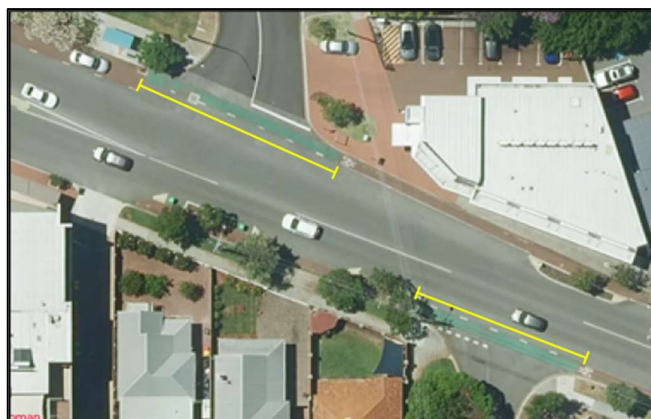
Figure 6.2 - Application of green surface treatment to a side road (Scarborough Beach Road, Mount Hawthorn)
