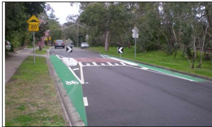
Figure 6.9 - Application of green surface treatment at one-way slow point bicycle bypass (Glen Iris, Melbourne)
