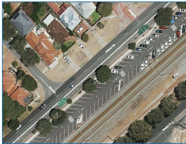
Figure 6.11 - Bicycle lane safety strip as part of Traffic Management Plan for Bayswater Station Upgrade (Railway Parade, Meltham)
