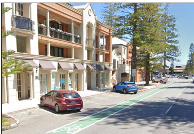
Figure 6.6 - Application of green surface treatment where a bicycle lane interfaces with angled street parking (Norfolk Street, Fremantle)
