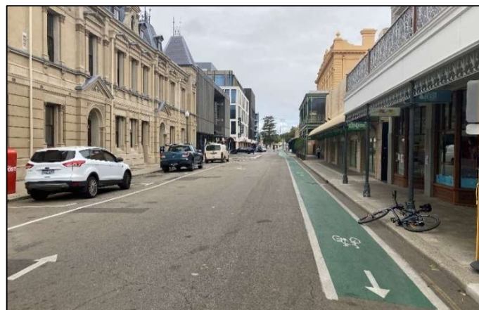
Figure 6.4 - Application of green surface treatment on contraflow bicycle lane (William Street, Fremantle)
