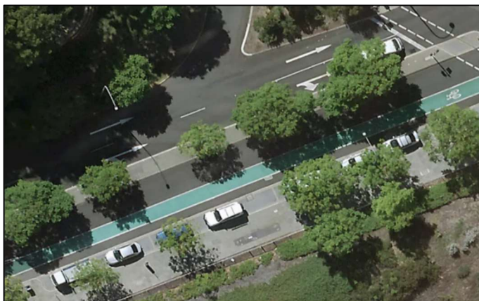
Figure 6.5 - Application of green surface treatment where a bicycle lane interfaces with parallel parking (Mount Street, Perth)
