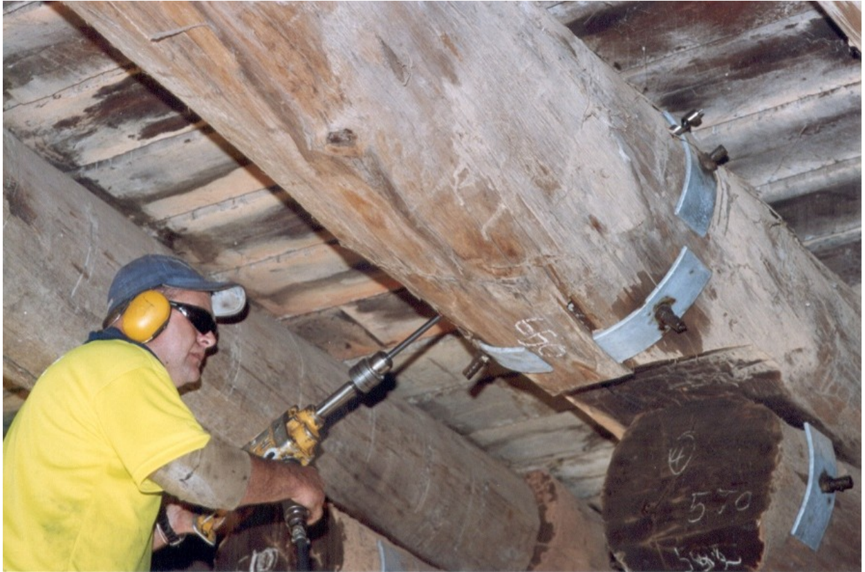
Maintenance of jarrah stringers – drilling reservoir hole for borate treatment.
