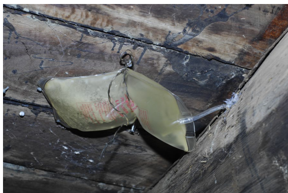
Reservoir bag in place. Note the need for care in positioning, to facilitate complete drainage.
