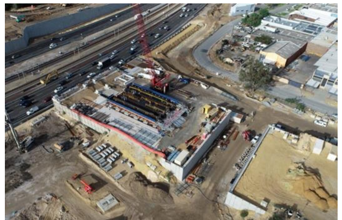
Stephenson Avenue Interchange Bridge casting launch bed.
