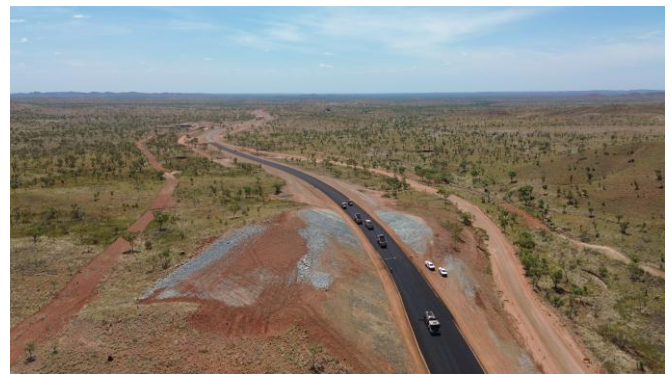
Recently reconstructed section of Tanami Road
