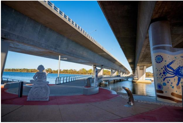
Yarning Circle Statues installed on the Mandurah Estuary Bridge
