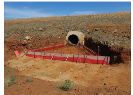
Apron formwork ready for concrete pour with completed road embankment.
