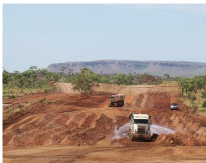
Constructing road embankment at SLK 38
